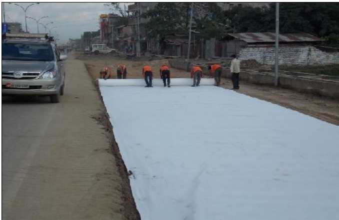
Laying of Nonwoven Geotextile TechGeo PR20 Fabric on subgrade
