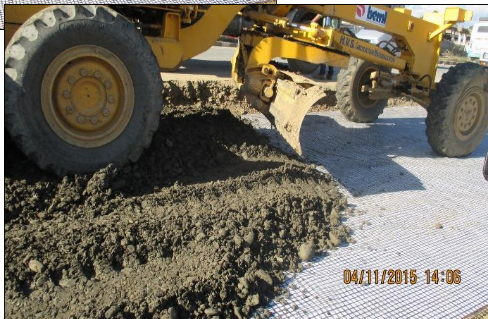
Laying of GSB on Geosynthetic Material
