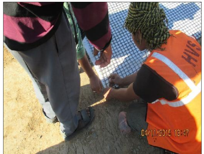
Levelling and fixing of Geosynthetic material on Subgrade
