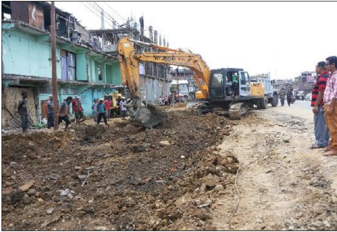
Preparation of sub-base for Road Expansion
