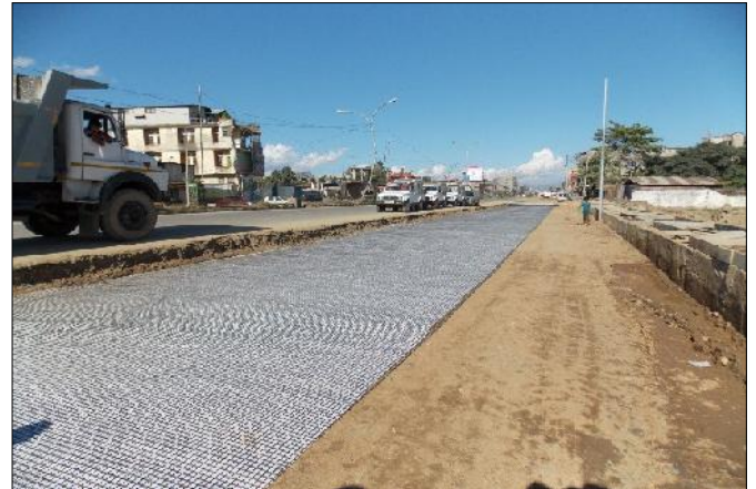
Laying of Biaxial Geogrid TFI TGB 30/20 on Subgrade
