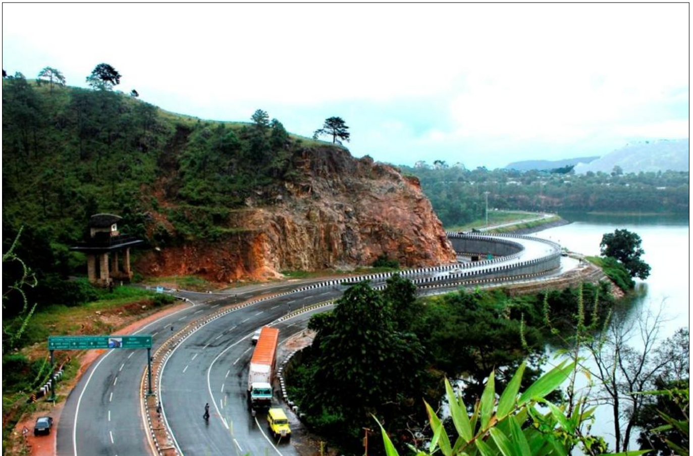
Before implementation of Rockfall Netting
