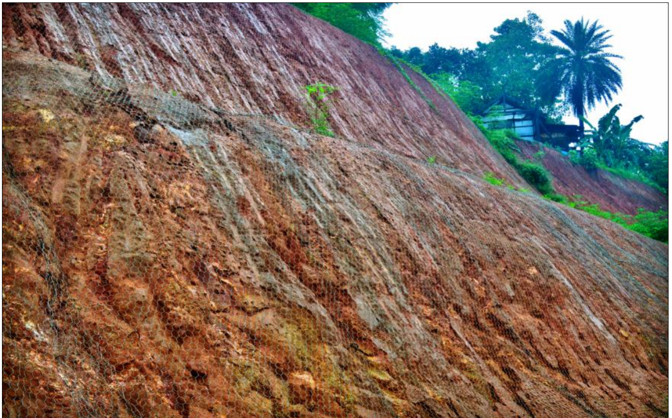
Slope after installation of Rockfall Netting
