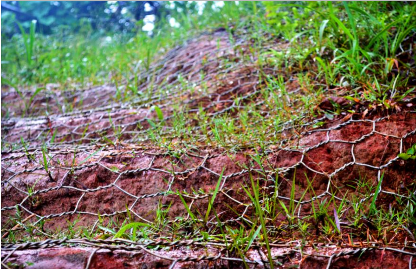
Top of Slope after Vegetation has grown
