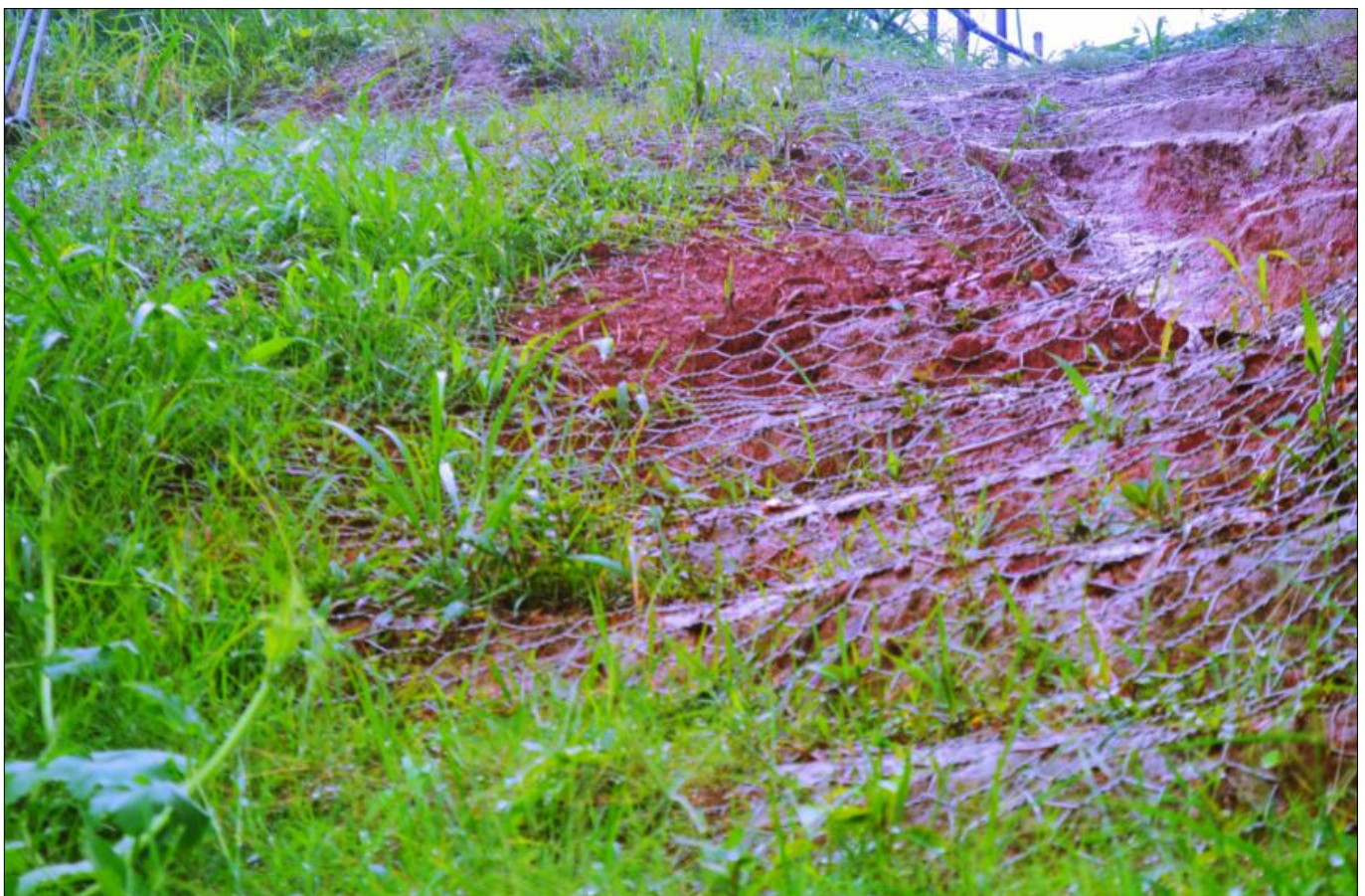
Top of Slope after Vegetation has grown
