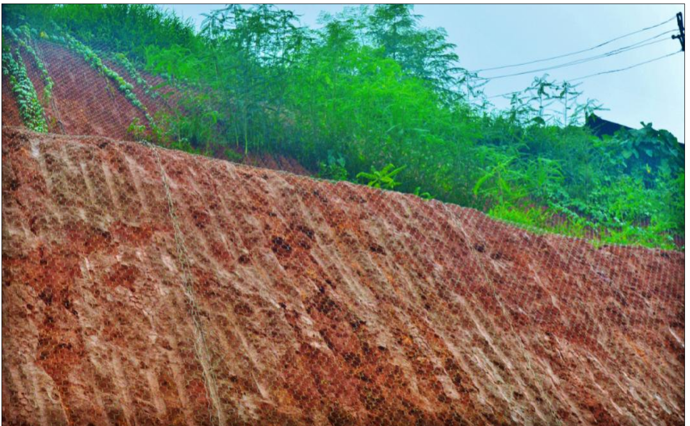
Slope after installation of Rockfall Netting
