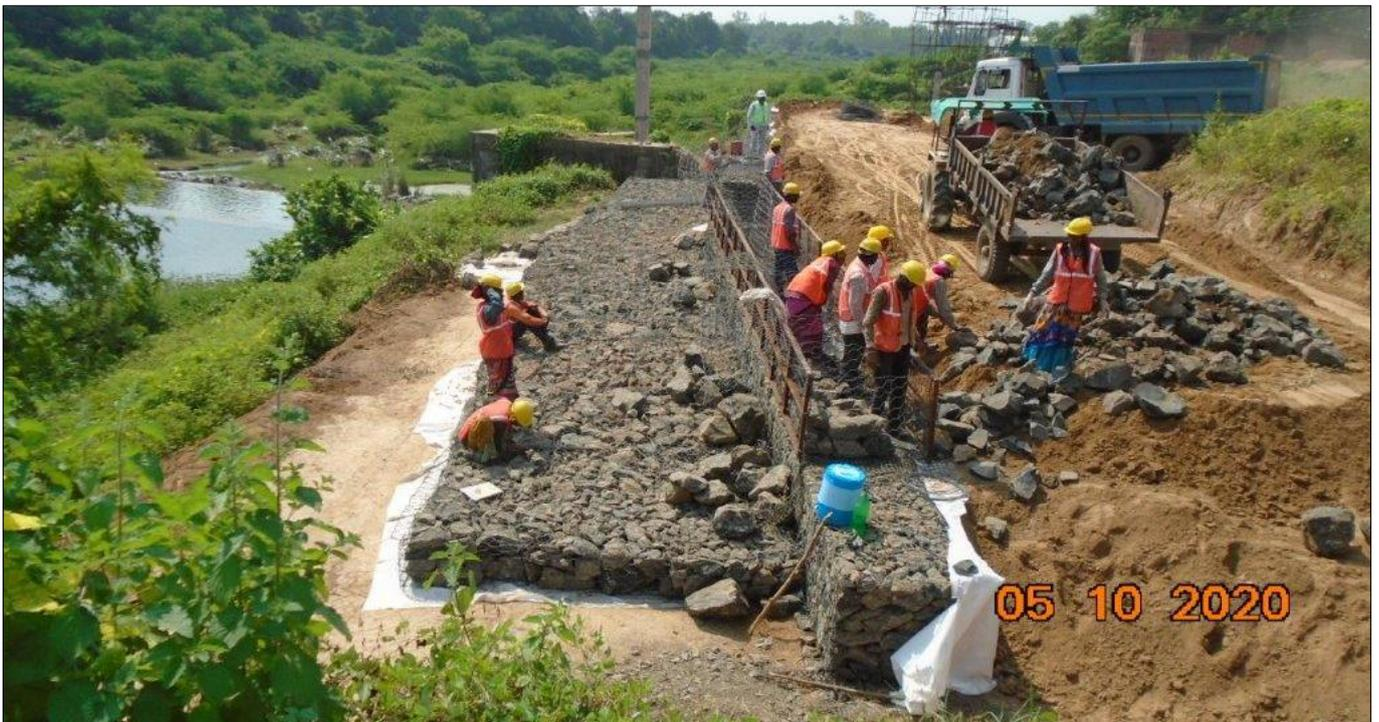
**Work under Construction - Gabion Facia & Mattress Installation**
