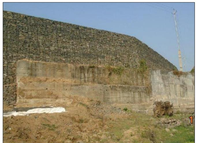
**Reinforced Soil Wall with Gabion facia**
