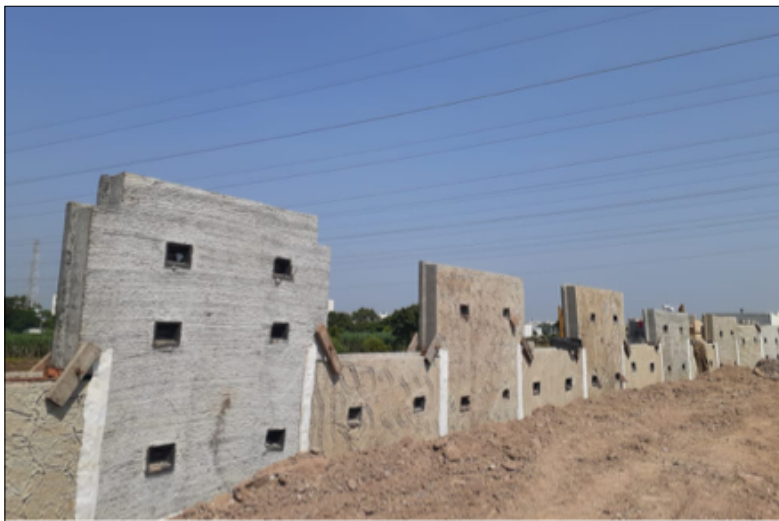
Erection of RCC Facia Panel in Progress
