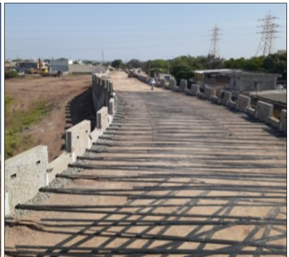
Installation of top layer TechStrap Polymeric Strip
