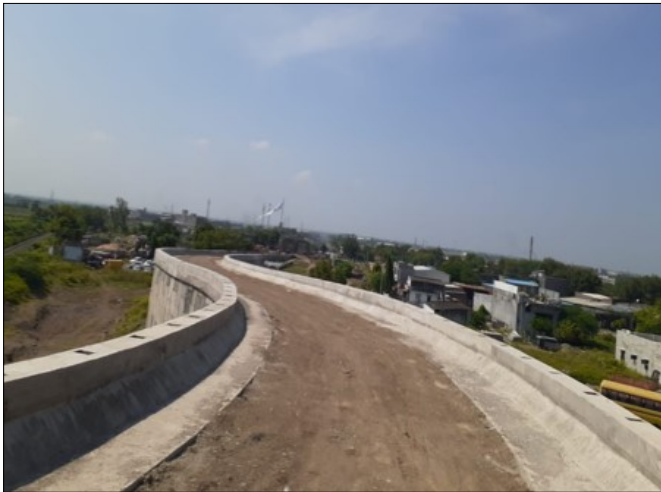
Coping beam installation completed
