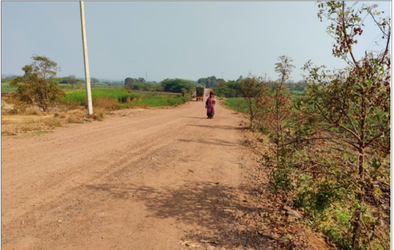
Pavement Subgrade Surface is Prepared for Laying of Drainage Composite
