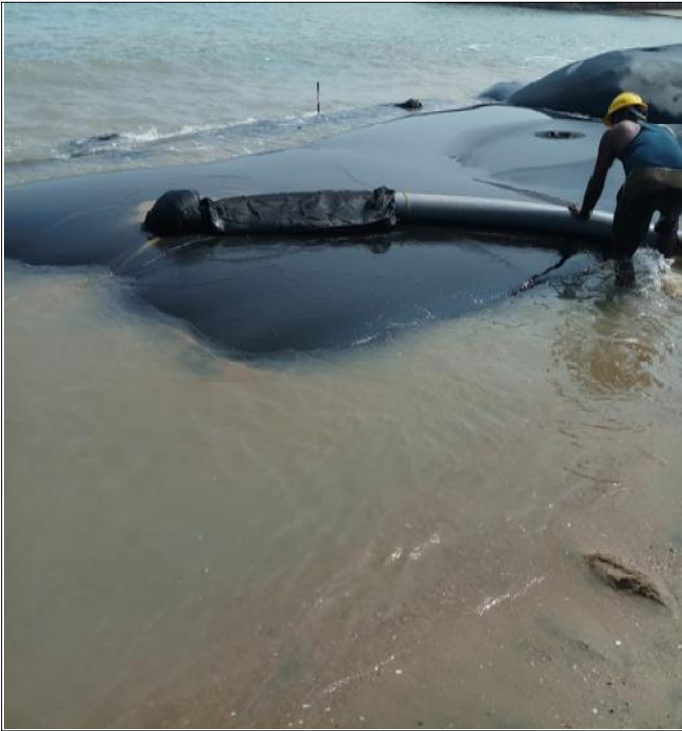
Geotextile Tube filling is in progress
