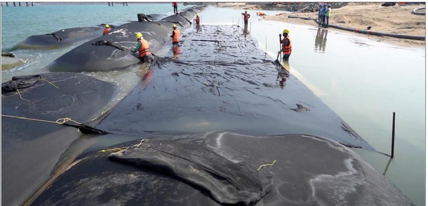
Aligning of 3rd Geotextile Tube in base layer is in progress
