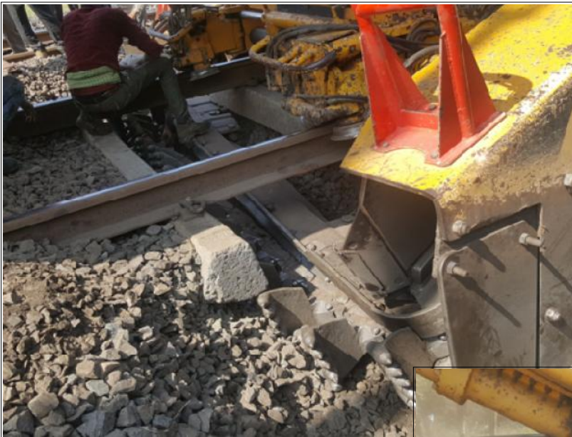
Removal of ballast with BCM machine in progress
