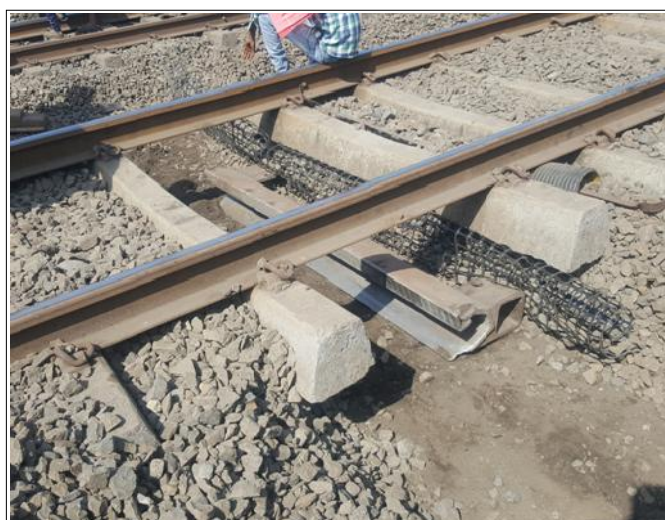
Placement of Sleeper Blade
