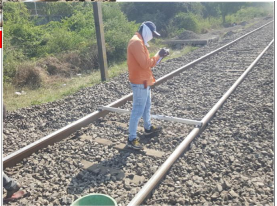
Measurement of gauge width after completion
