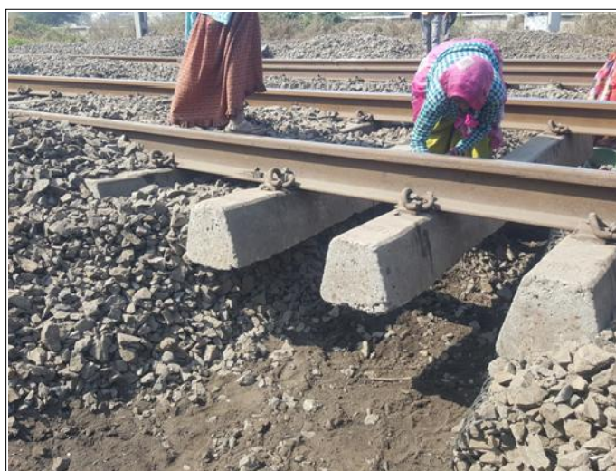
Manual Removal of Ballast in Progress
