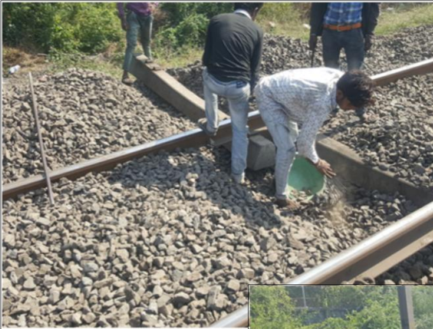
Placement of sleeper back to position
