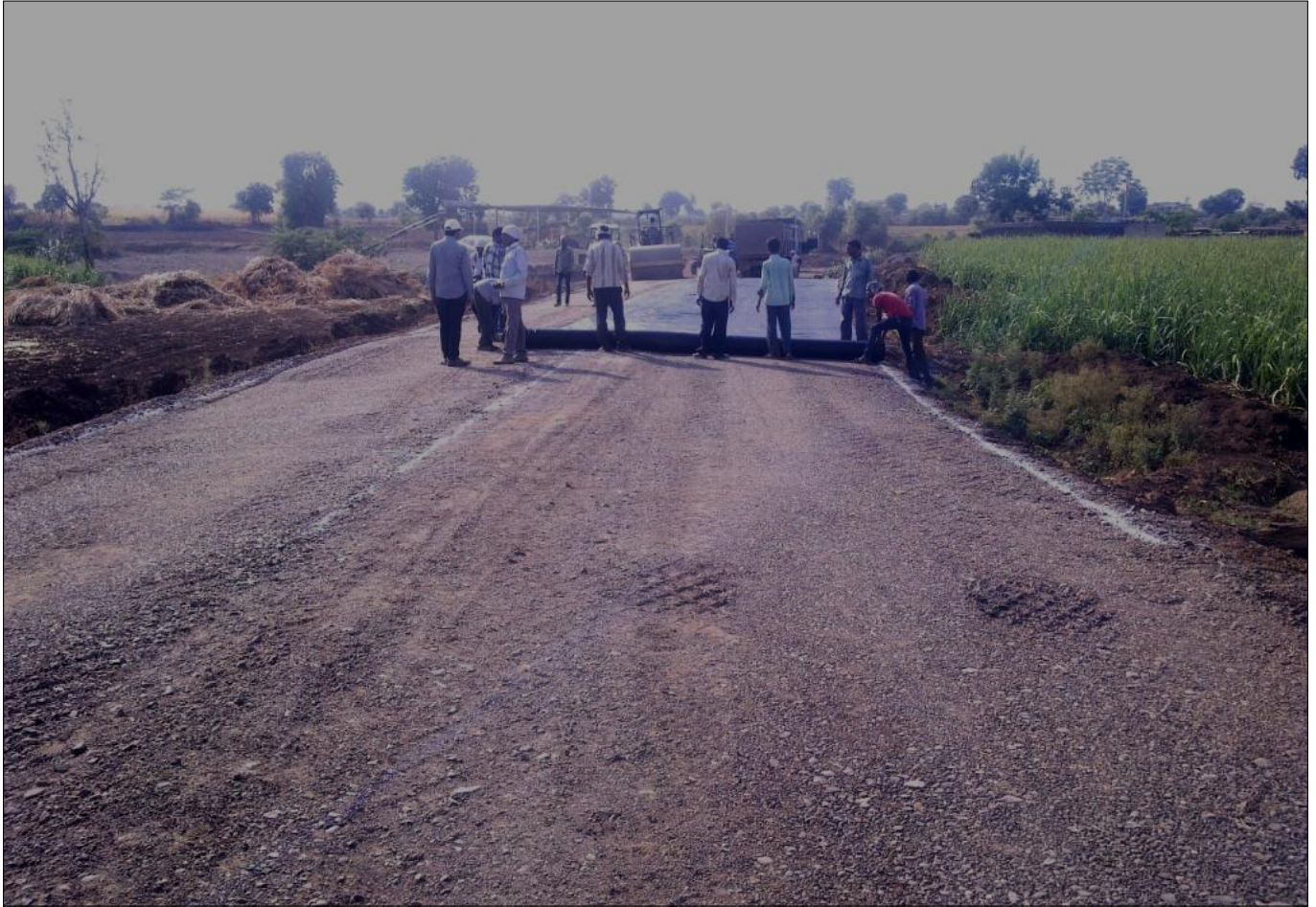
Photo 7 : Laying of woven Geotextile TFI - 5300 Type-1
