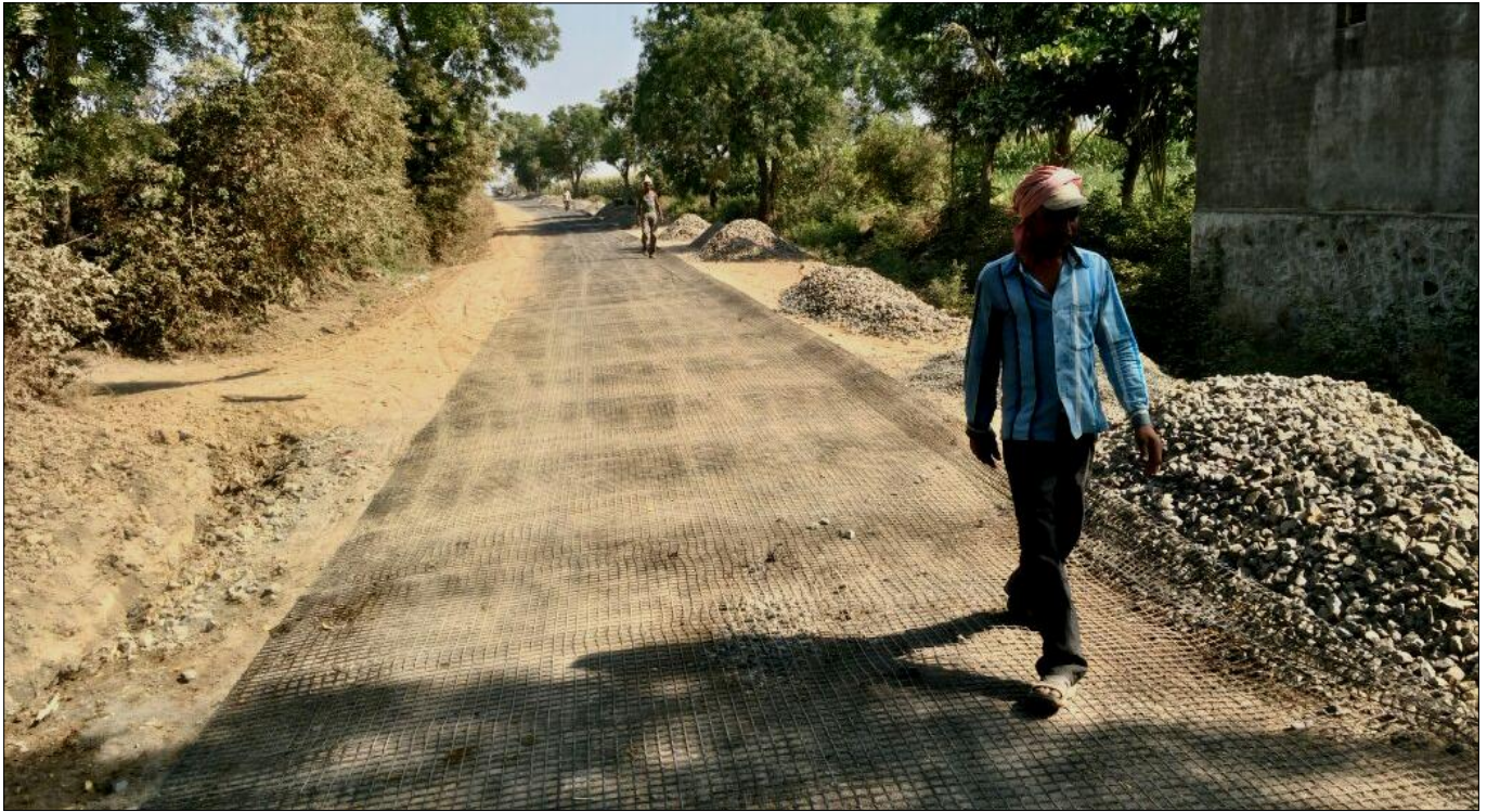
Photo 9 : Laying of TechGrid Geogrid TGB-40
