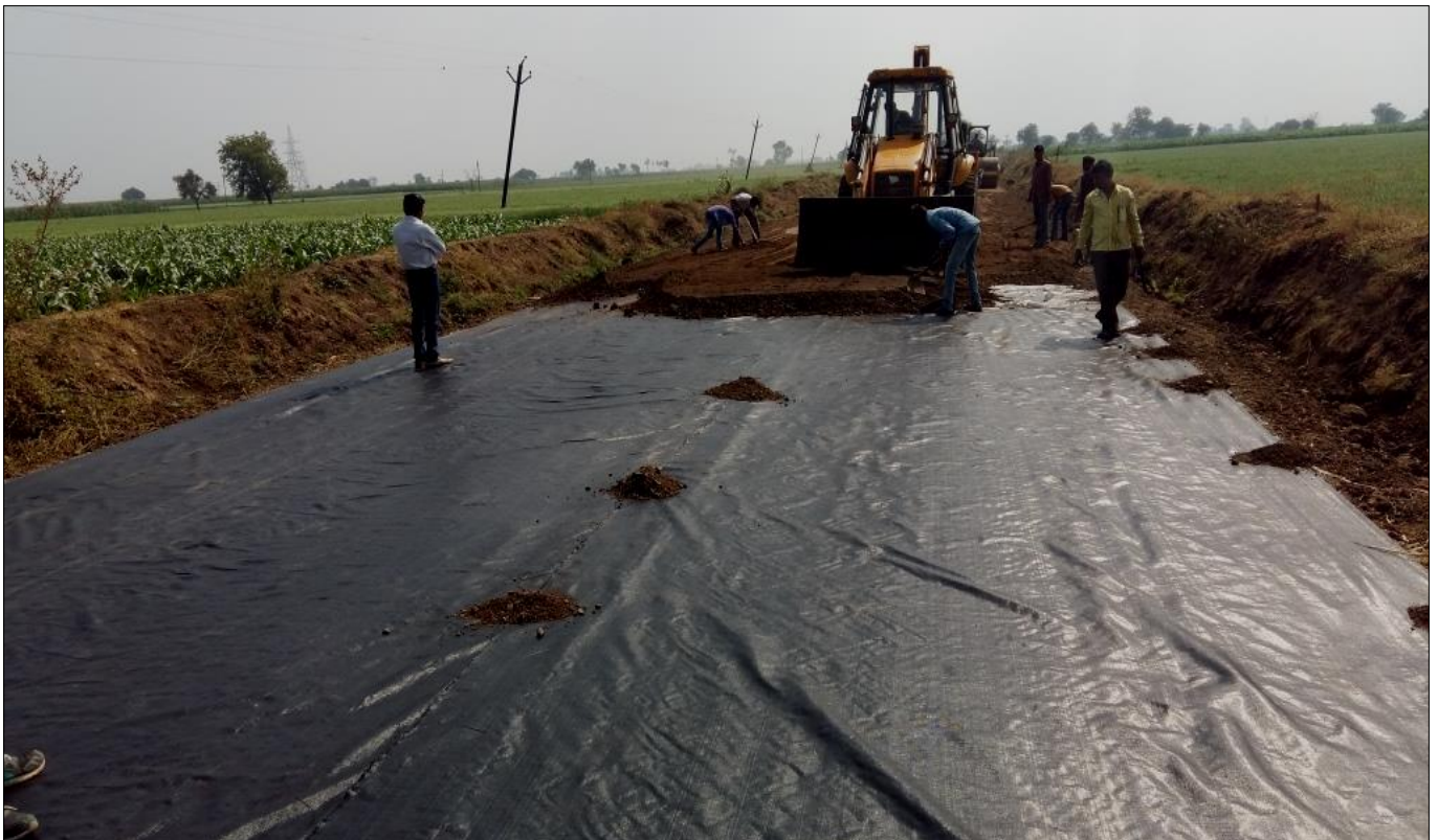
Photo 8 : Placing of Sand over Woven Geotextile TFI - 5300 Type-1
