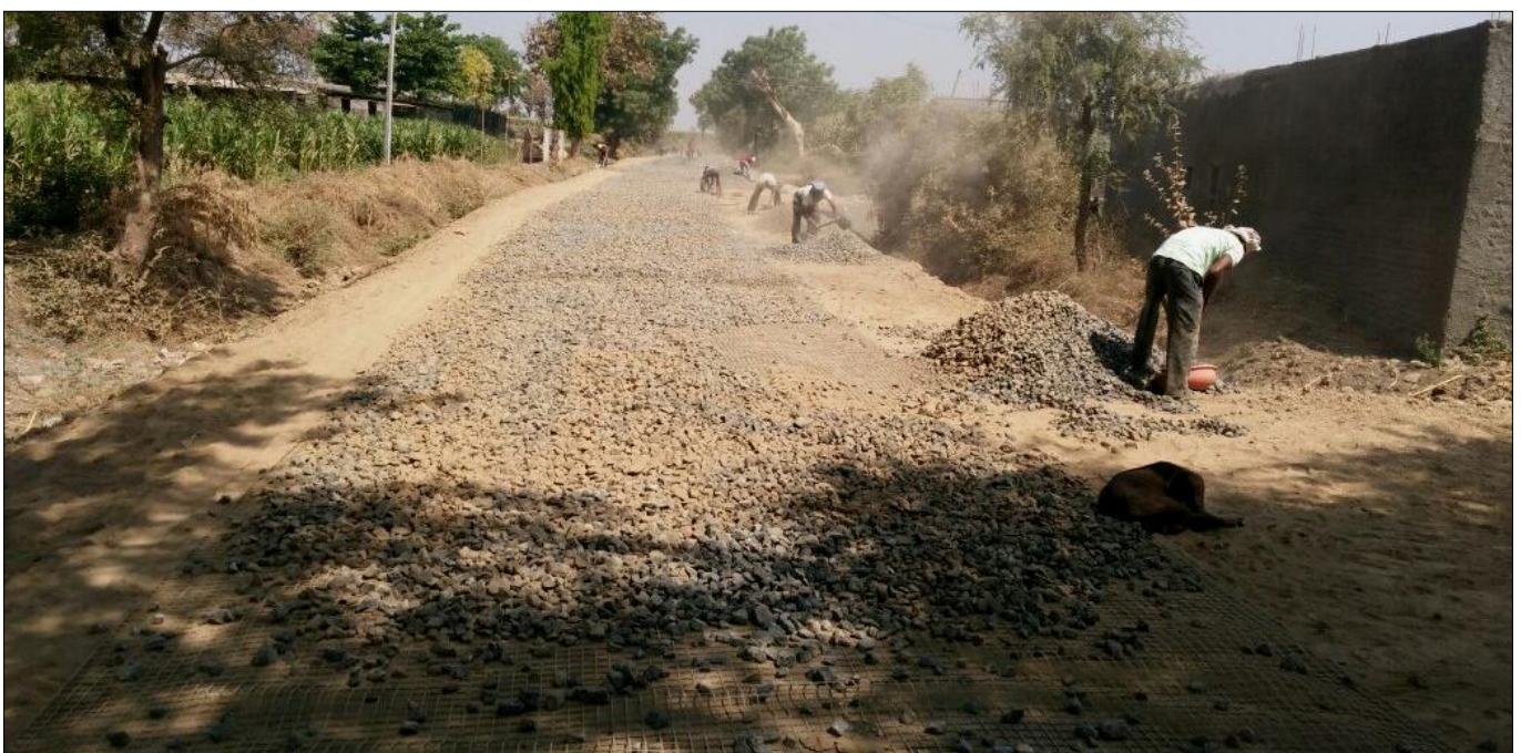
Photo 10 : Placing of MPM over TechGrid Geogrid TGB-40
