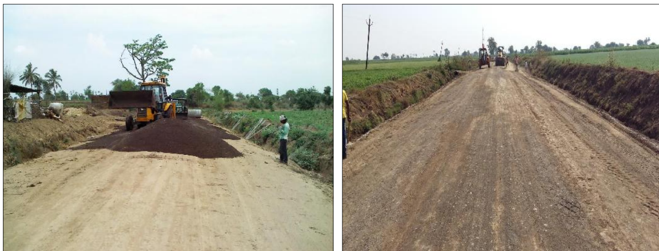
Photo 4 & 5 : Sand Layer laid on prepared surface
