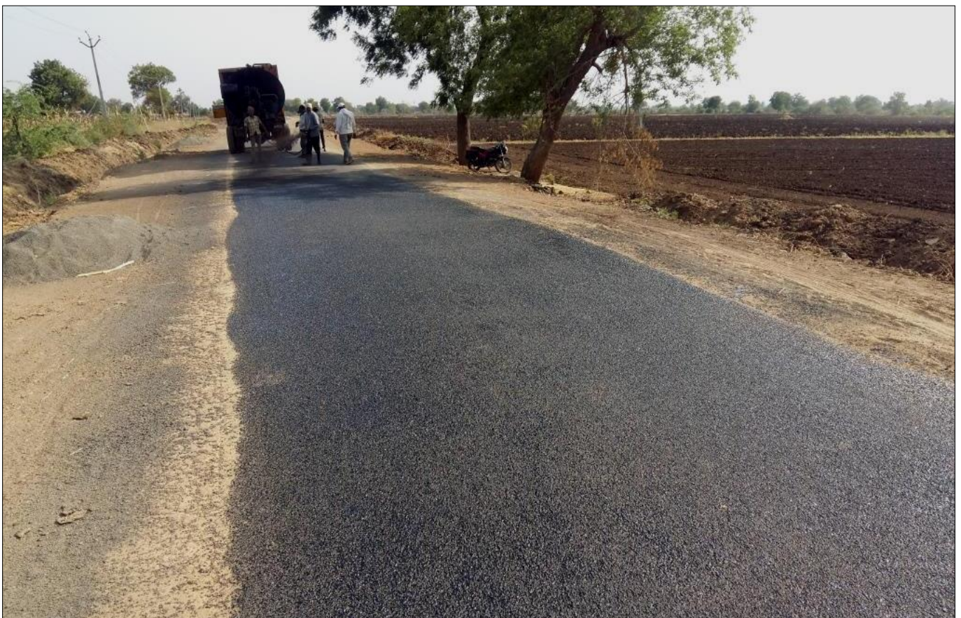
Photo 12 : Laying of Seal coat
