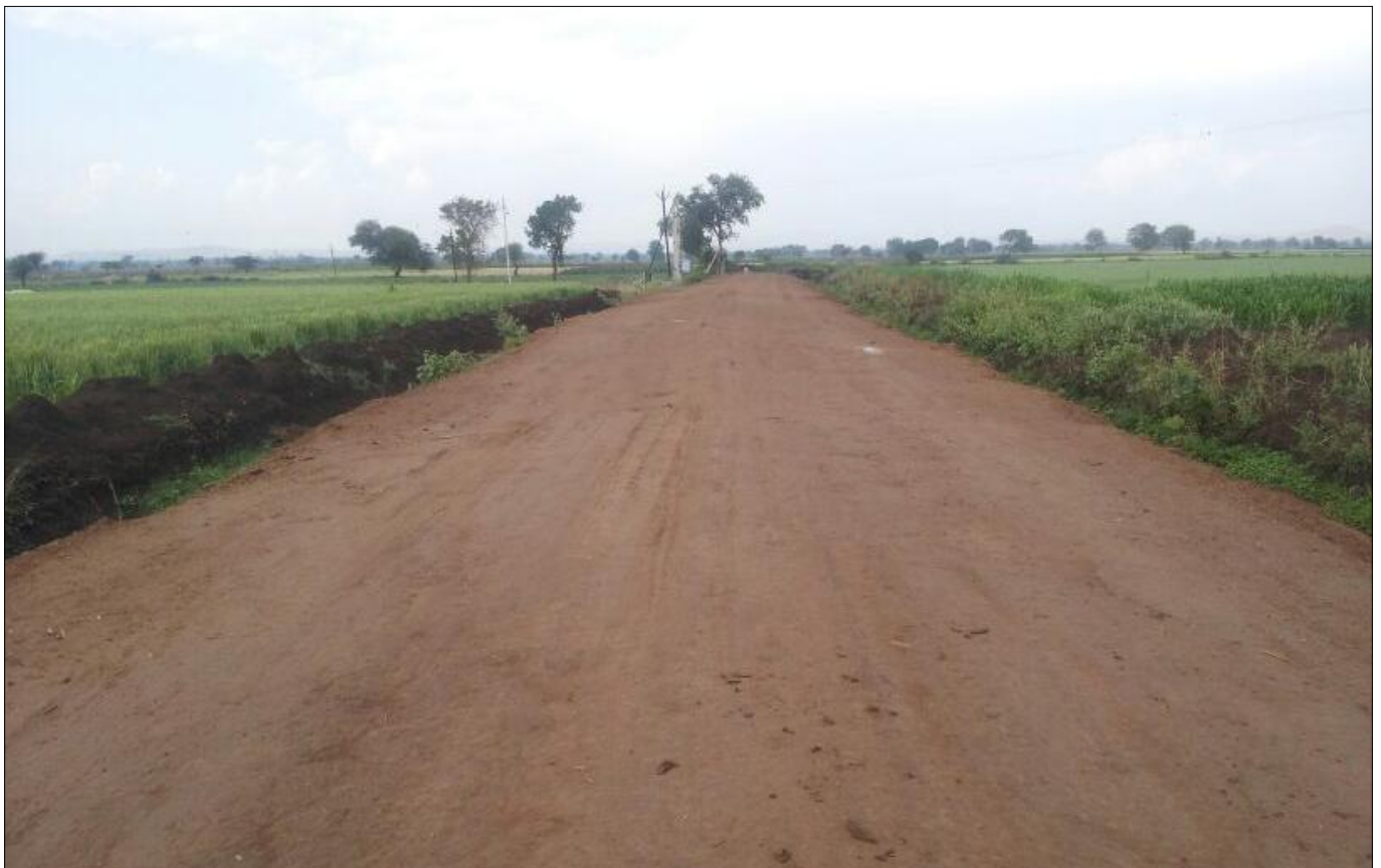
Photo 3 : Pavement Subgrade Surface is Prepared
