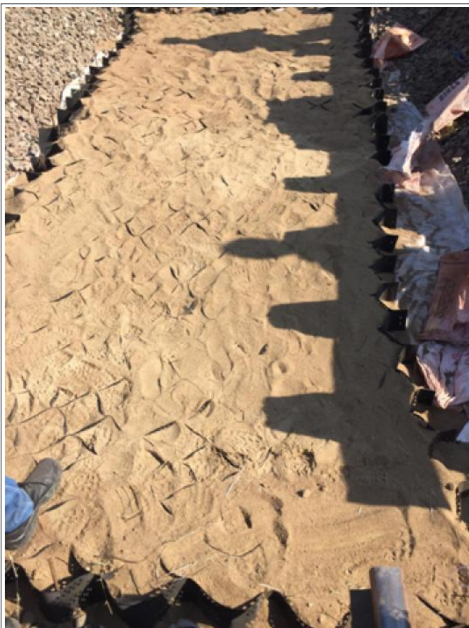
Filling of Techcell Geocell in Progress
