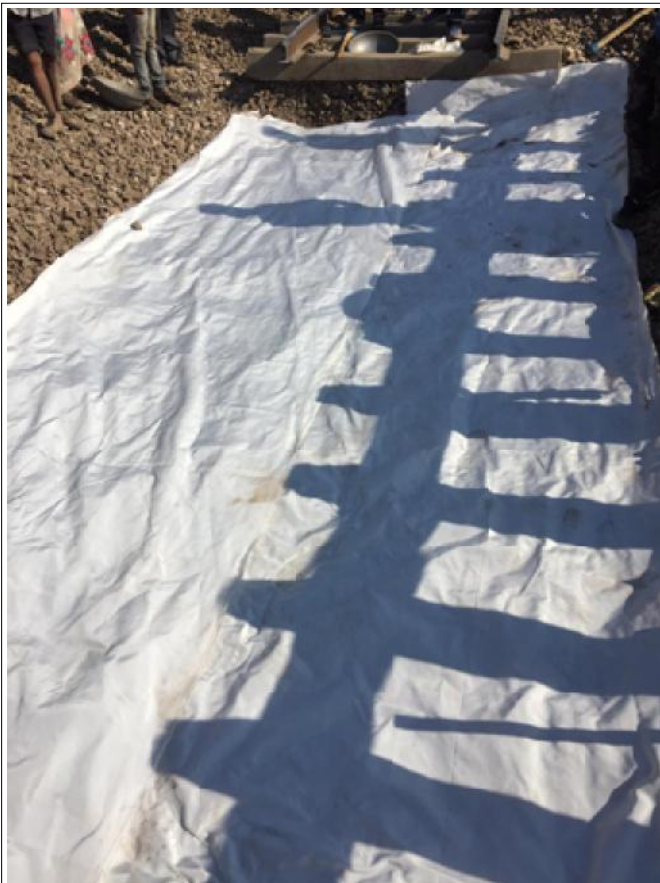
Laying of Woven Geotextile
