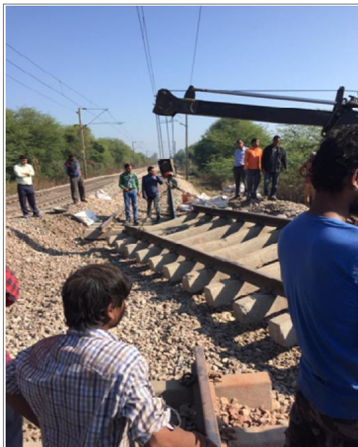
Removing another track panel
