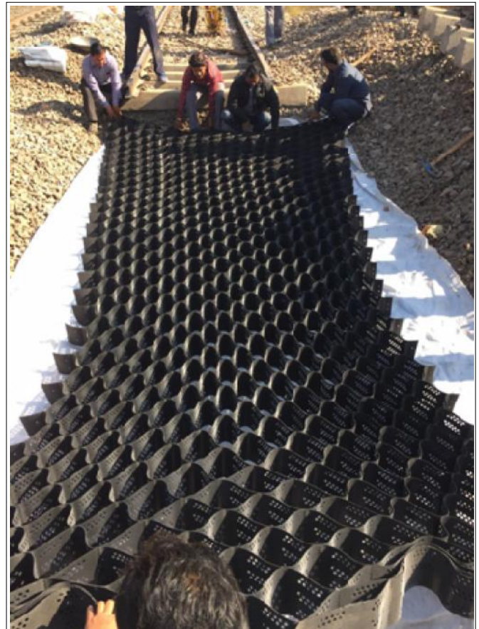
Laying of Techcell Geocell in Progress
