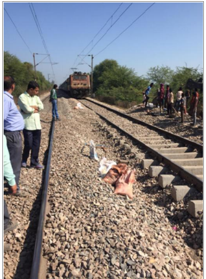
After laying of track in completed stretch
