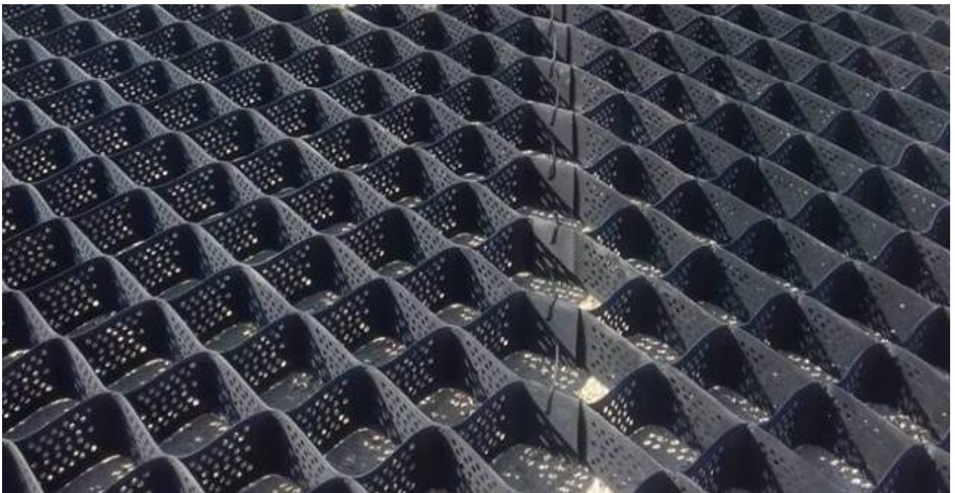
Joining of two Geocells with Cable Ties
