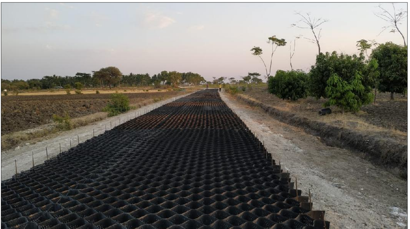
Spreading of TechCell Geocell above the subgrade
