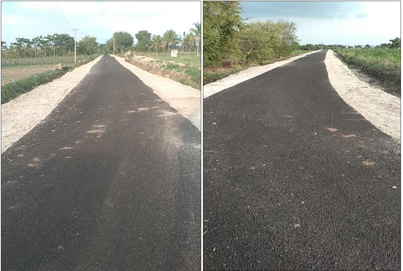
Road Pavement after completion
