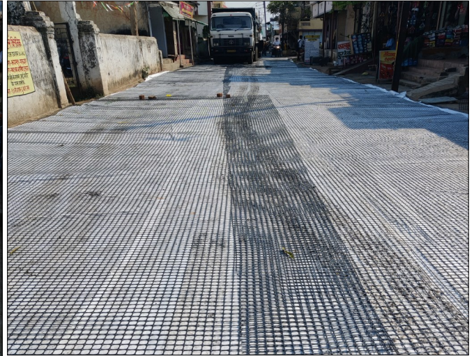
Photo 2 : Laying of PP Biaxial Geogrid over TechPave
