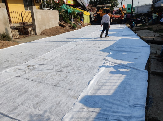
Photo 1 : Laying of TechPave C040
