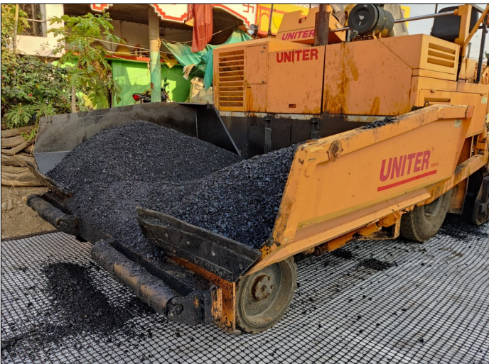
Photo 3 : Placing of Asphalt mix over PP Biaxial Geogrid
