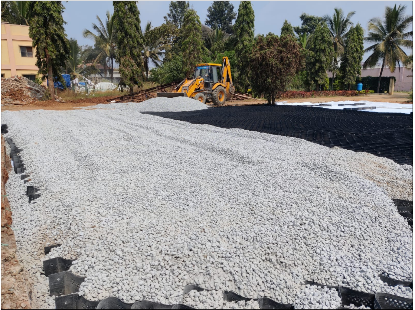
Photo 6 : Filling of Techcell Geocell with GSB
