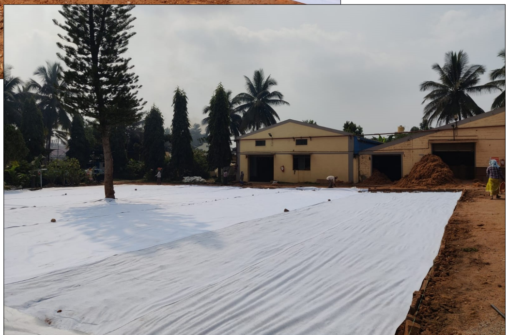
Photo 2 & 3 : Installation of TechGeo Nonwoven Geotextile
