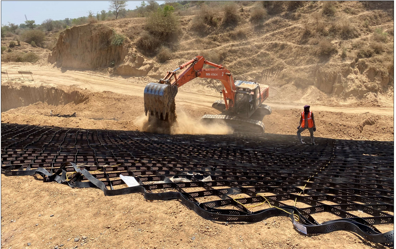
Photo 2 : Filling of vegetative soil in Techcell Geocell
