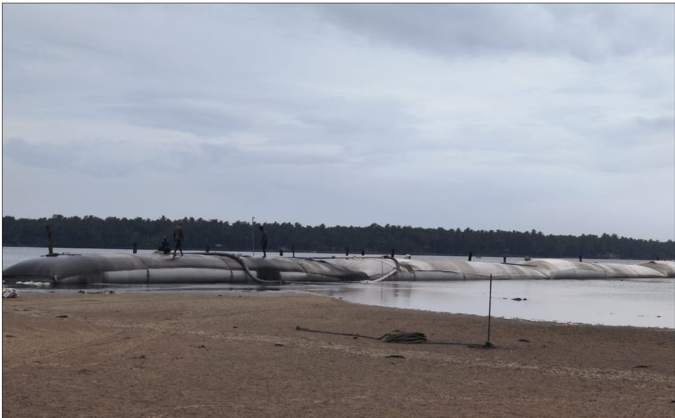
During Construction Photographs
