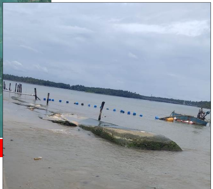
Damaged existing Geotextile Tubes
