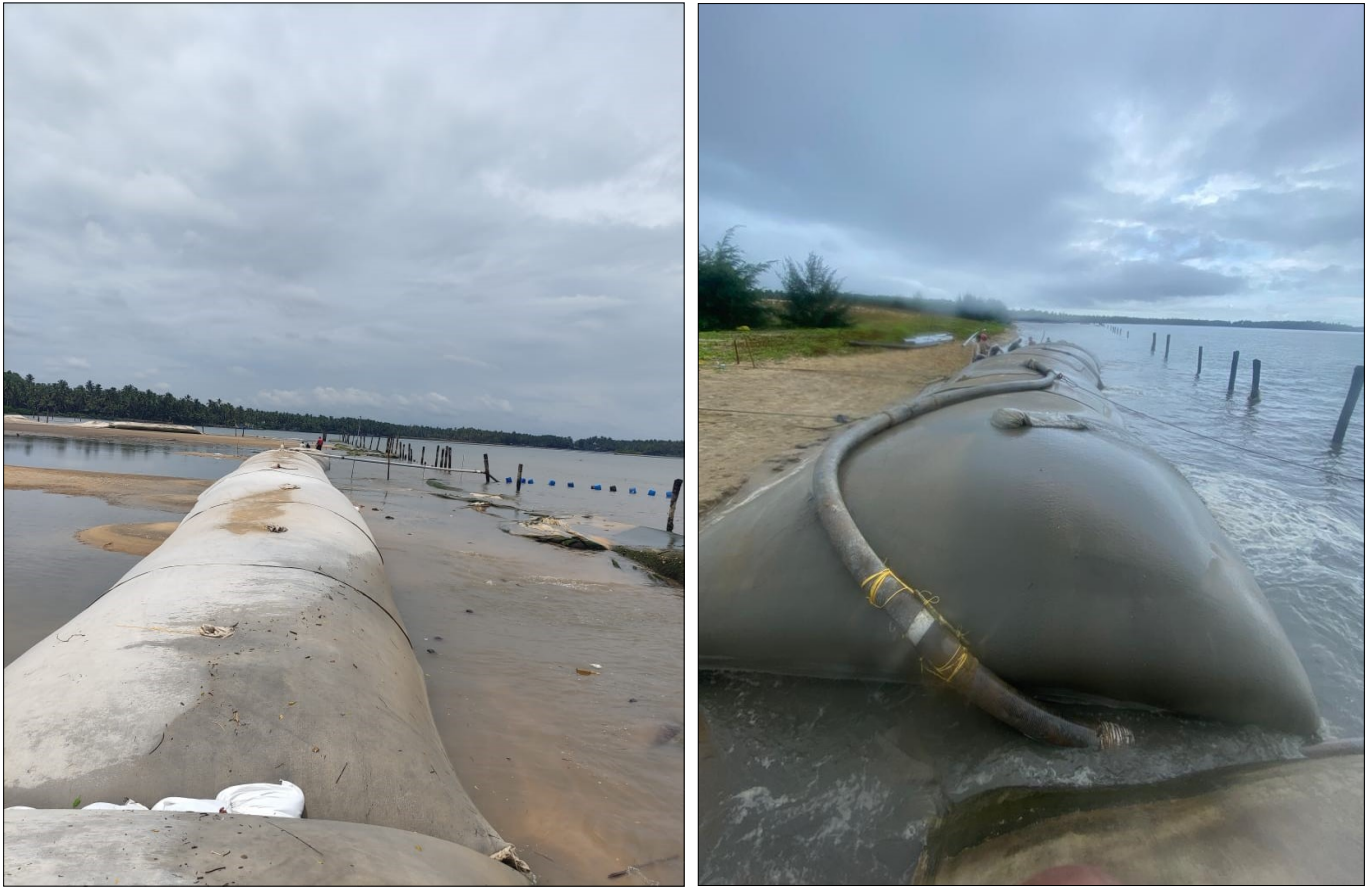
After Construction photographs
