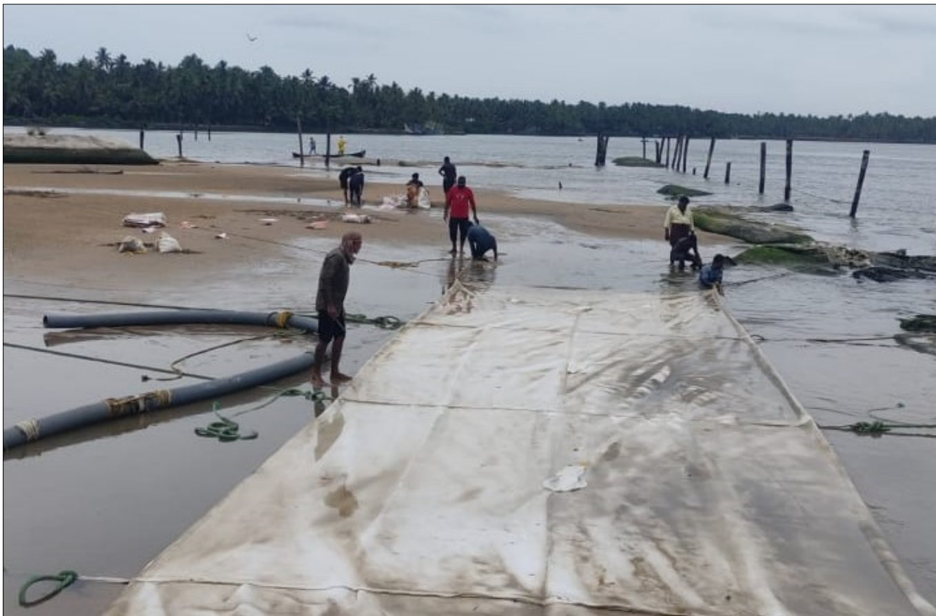
Laying of TechTube Geotextile Tubes in progress
