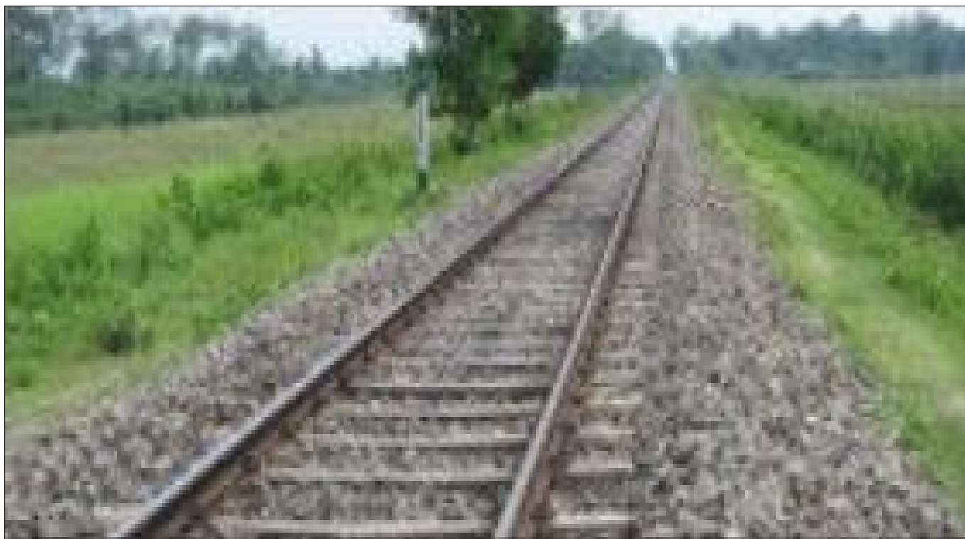
Photo 11 : Condition of the track two years after rehabilitation (as on June 2008)
