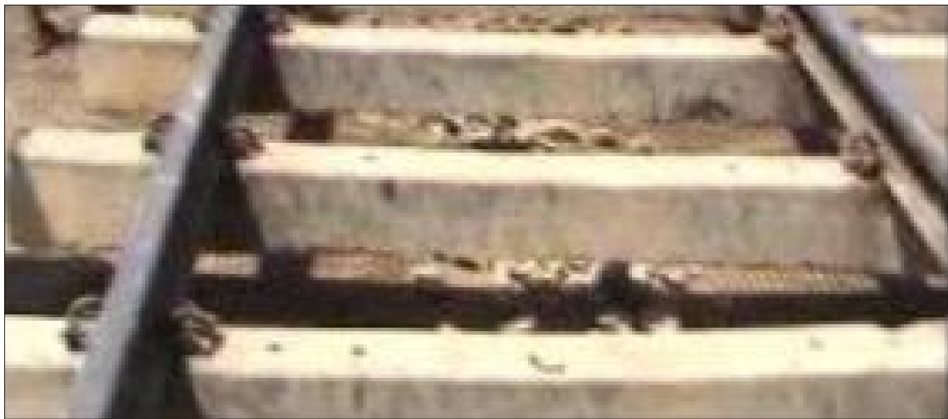
Photo 9 : Placing ballast over the geogrid
