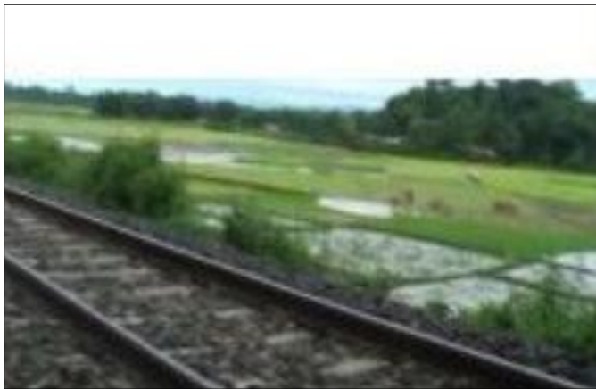
Photo 1 : Site before rehabilitation
