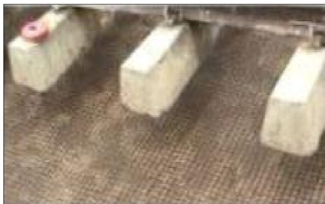
Photo 8 :Laying Techgrid TGB-40 Knitted Polyester Biaxial Geogrid
