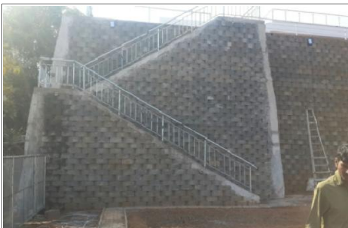
Fig 4 : After Construction of stairs
