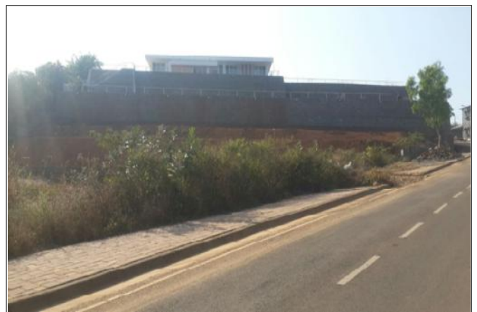
Fig 5 : After Construction - View from far
