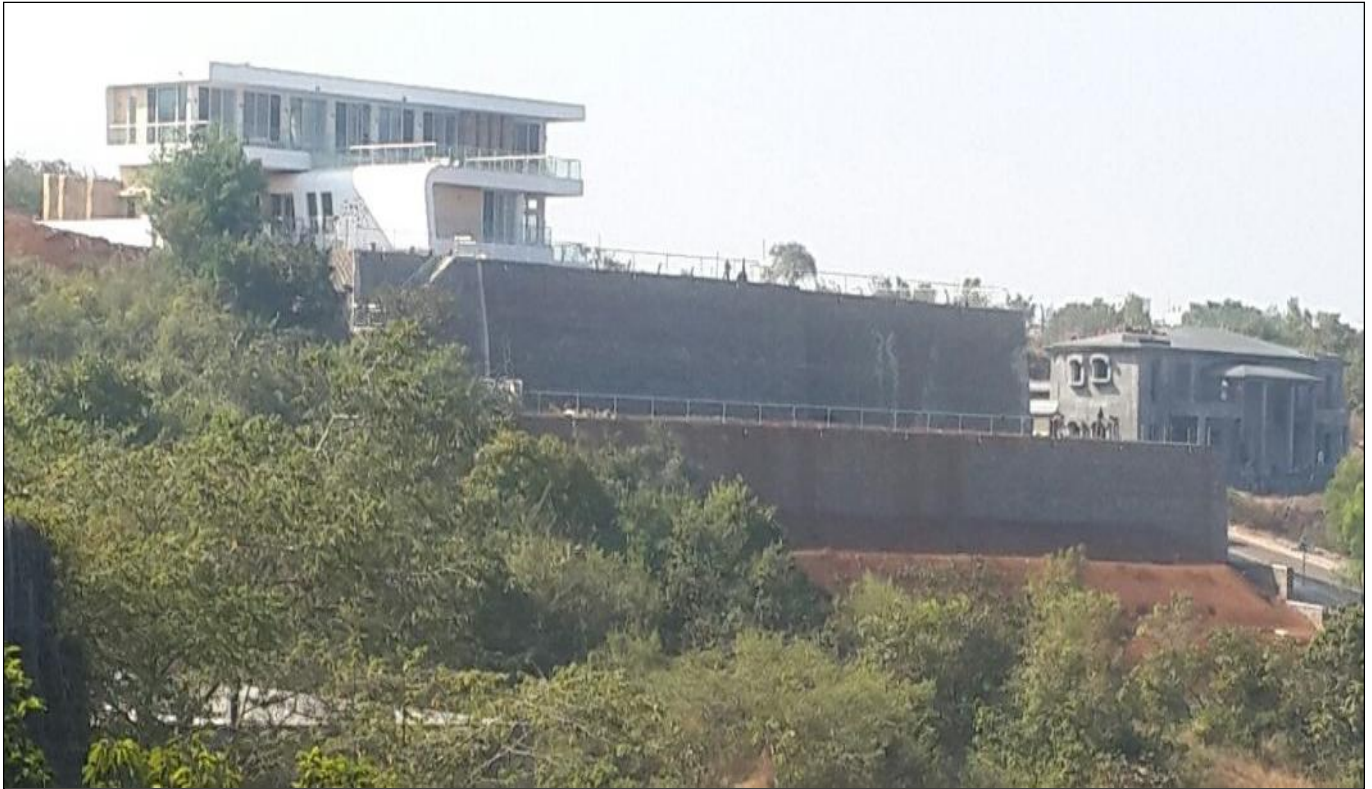
Fig 6 : Structure after Construction
