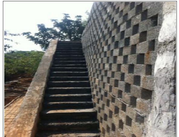
Fig 2 : Stairs over reinforcement
