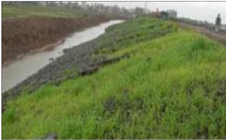
Embankment work in progress & partially completed
