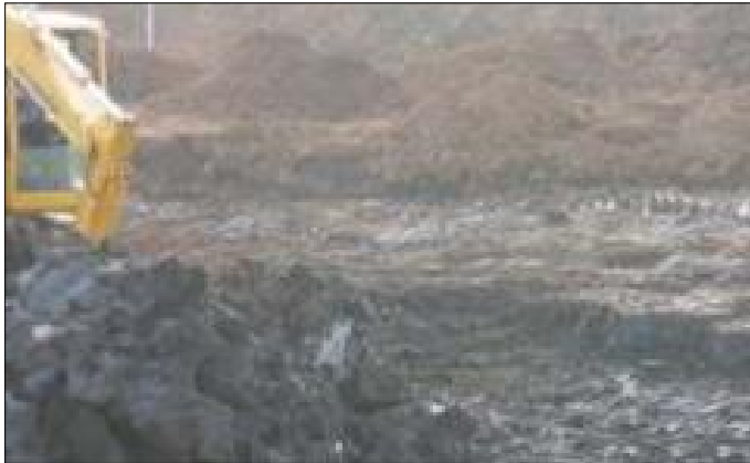
Existing Area Being Prepared
