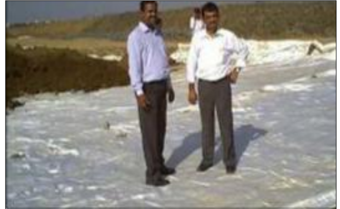
Laying of High Strength Geotextile TFI 3200
