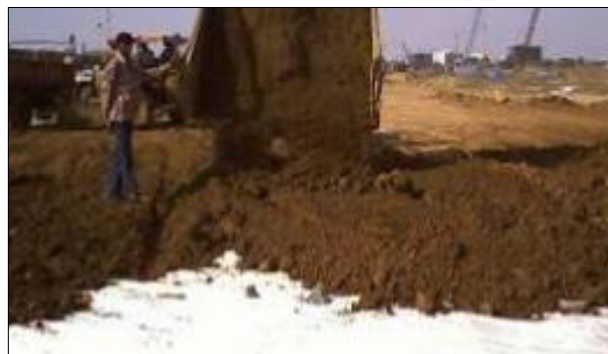
Murum Layer Being placed over Geotextile
