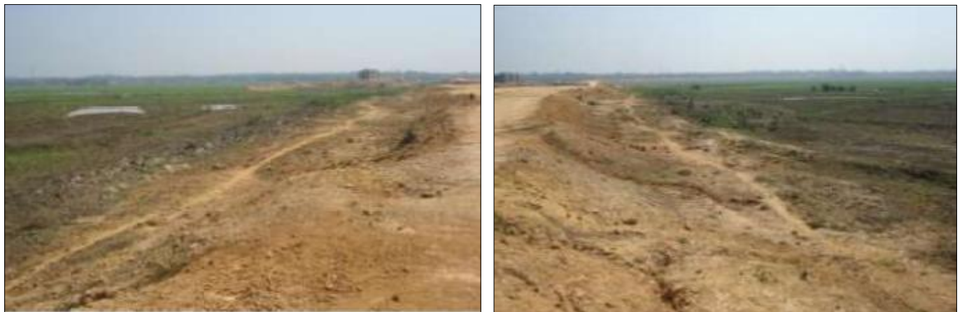
Figure 1 : Left and Right side of the Embankment
