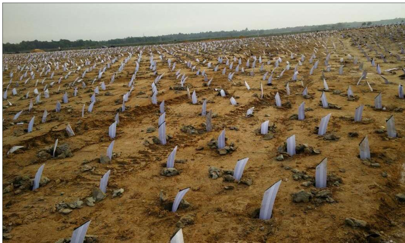
Installation of PVD
