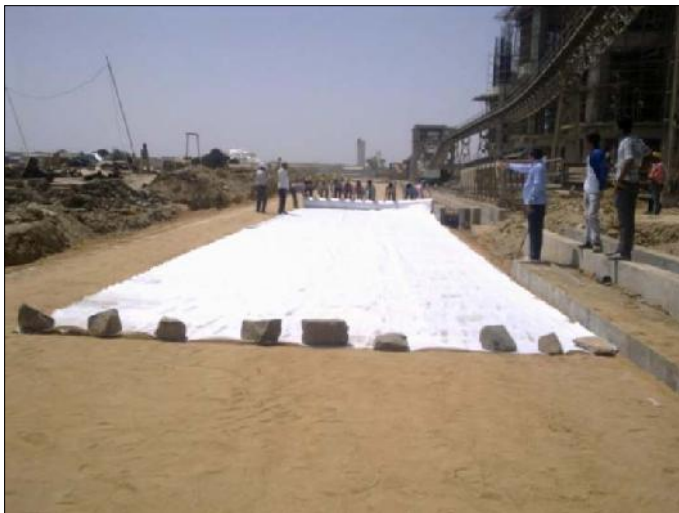
Fig 4 : Laying of TechGeo PR-20 (Non-Woven Geotextile)
