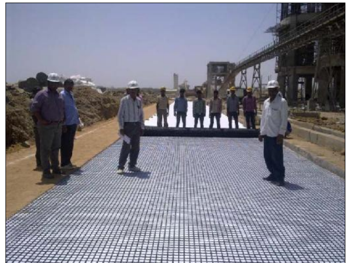
Fig 5 : Laying of TFB-40 over TechGeo PR-20
