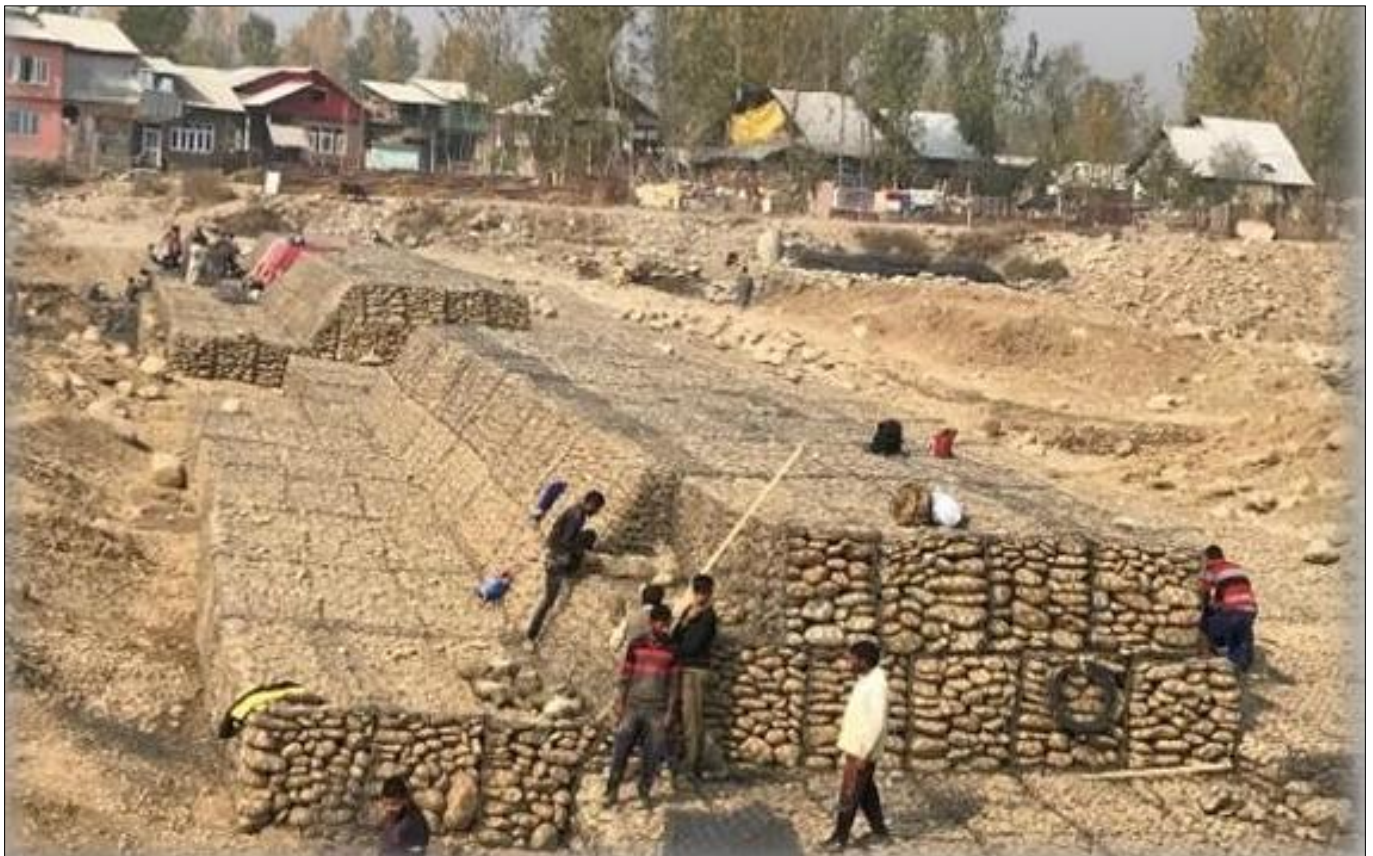
Photo 1: Gabion Installation in progress
