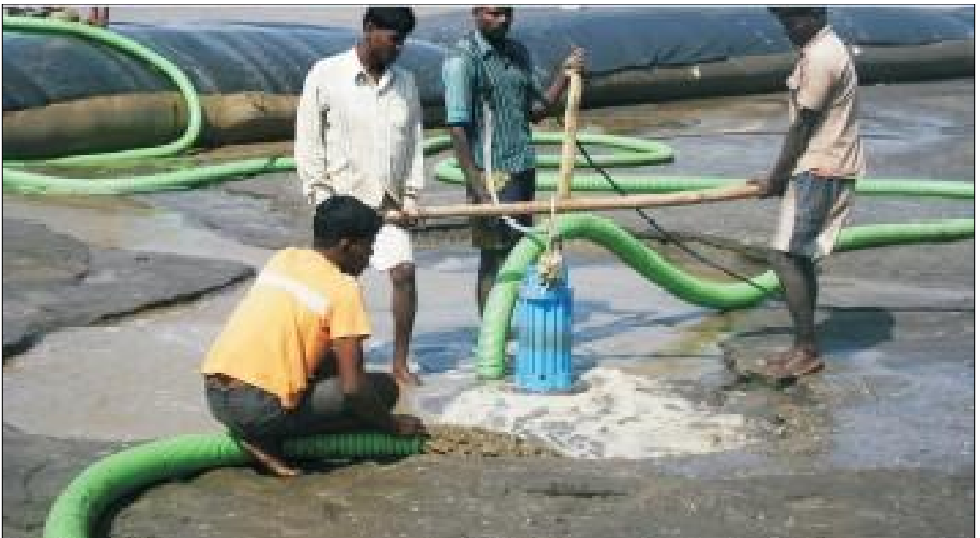
During Installation of TechTube
