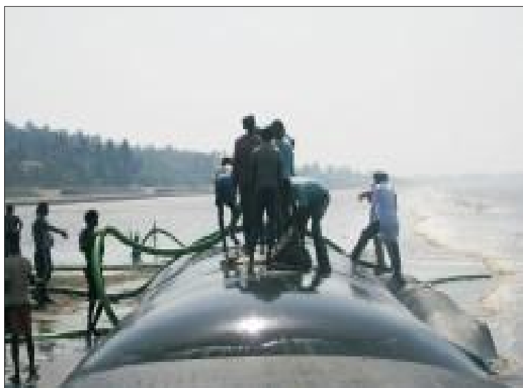
Installation of TechTube
