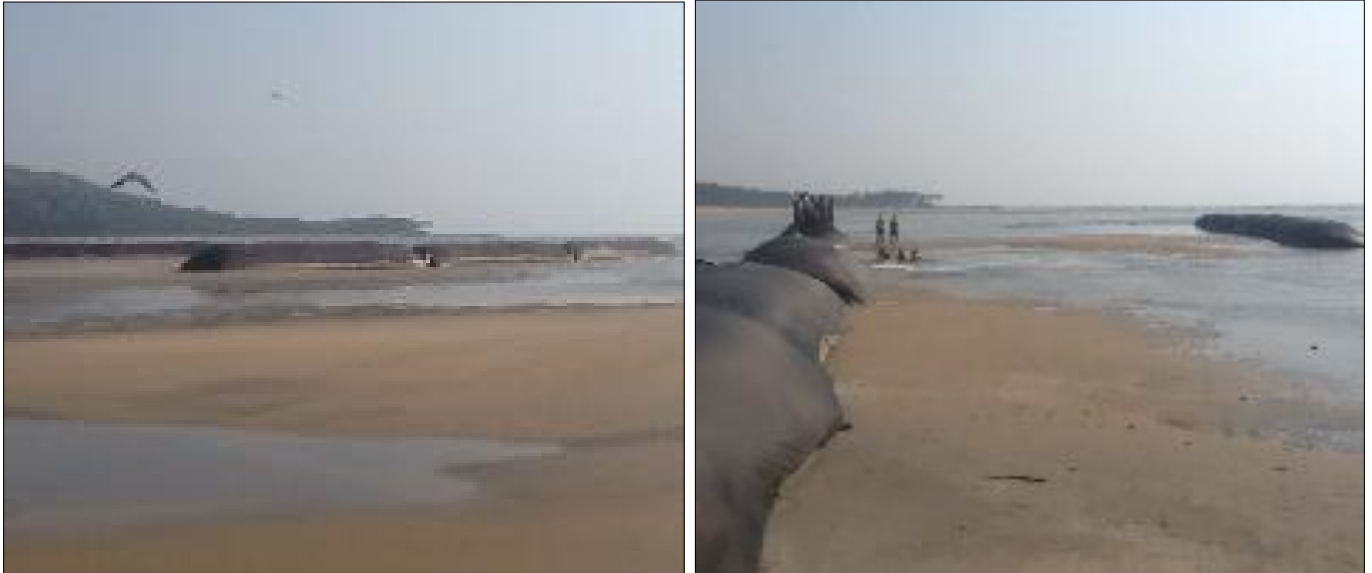
TechTubes At Devbagh Beach
