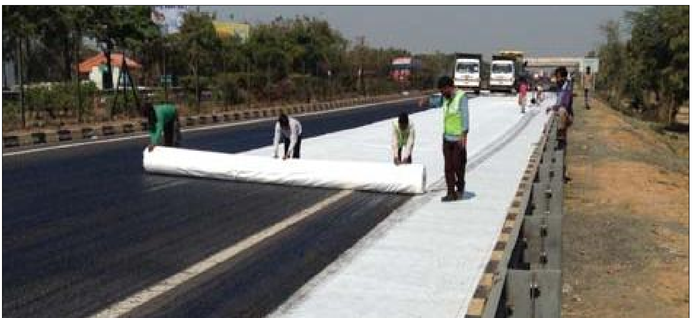
TechFab Paving Fabric - Installation
