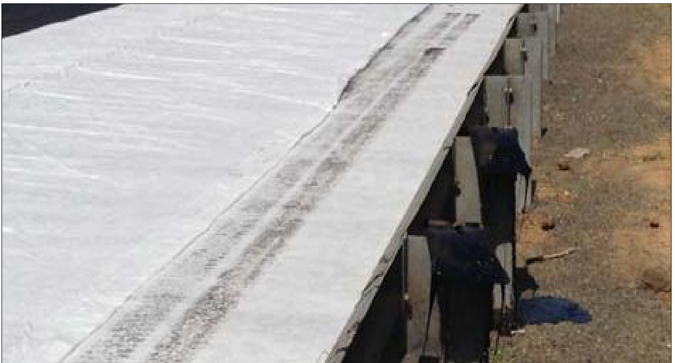
Installed TechFab Paving Fabric
