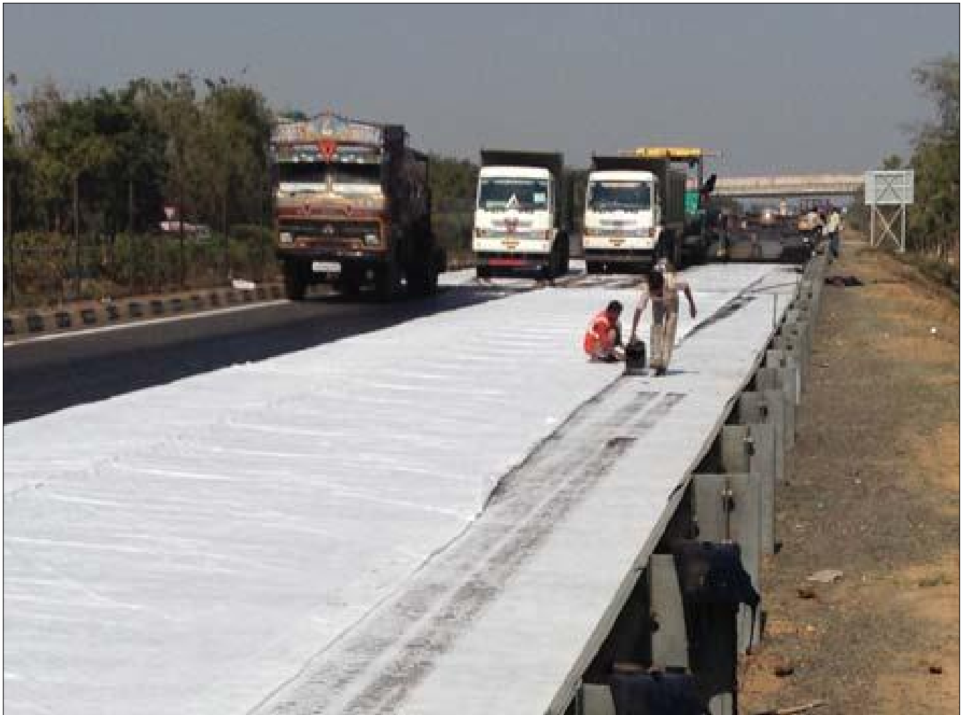
TechFab Paving Fabric - Installation
