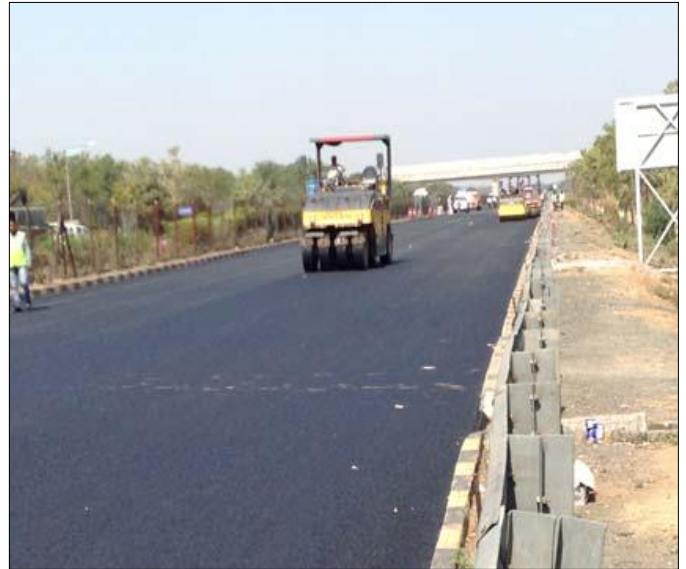
Compaction after placement of Overlay
