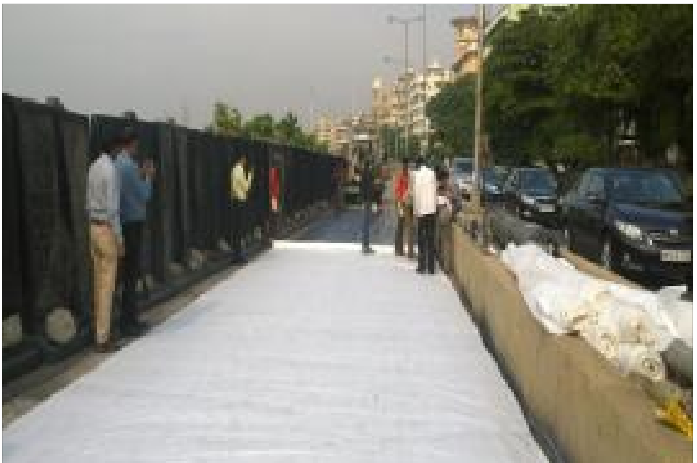
Installation of TechPave
