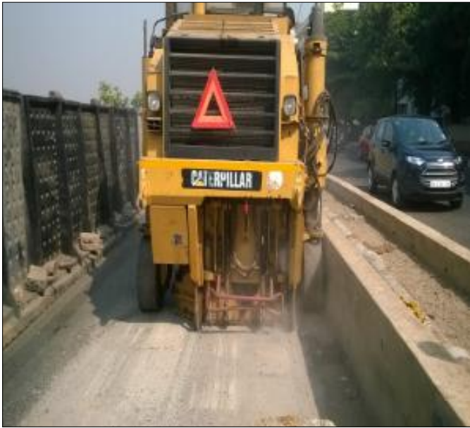
Milling Operation – Before Installation
