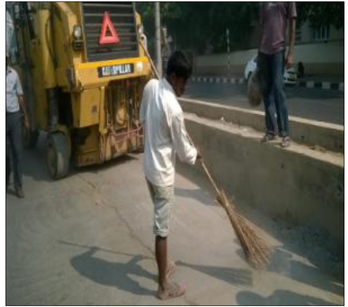
Surface Preparation Before Laying TechPave
