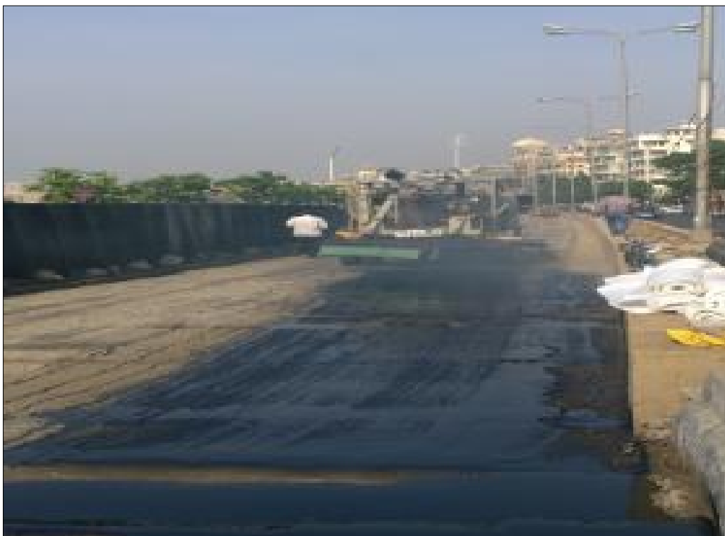
Spraying of Bitumen – Before TechPave
