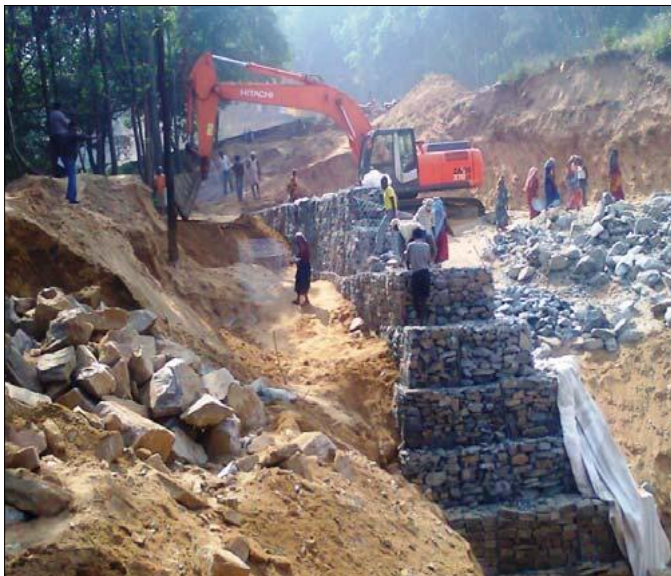
Photo 1 & 2 : TechFab Metal Gabion Installation in progress
