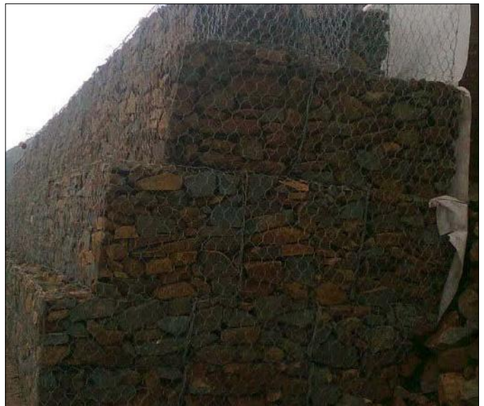
Photo 3: TechFab Metal Gabion Wall - Side View
