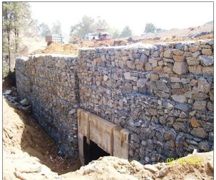
Photo 1 & 2 : TechFab Metal Gabion Installation in progress
