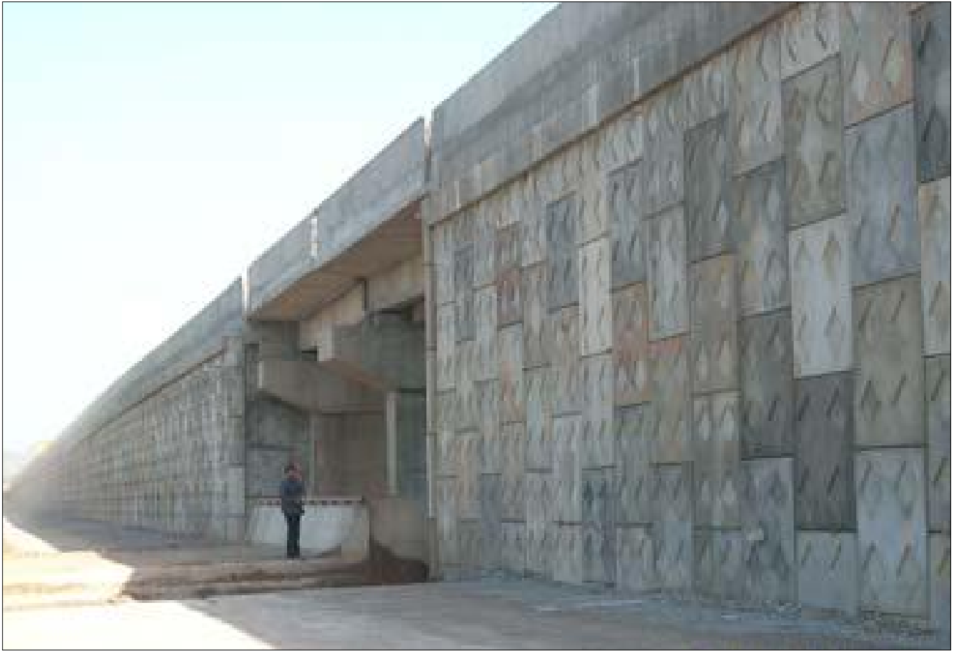
Elevation view of RS wall
