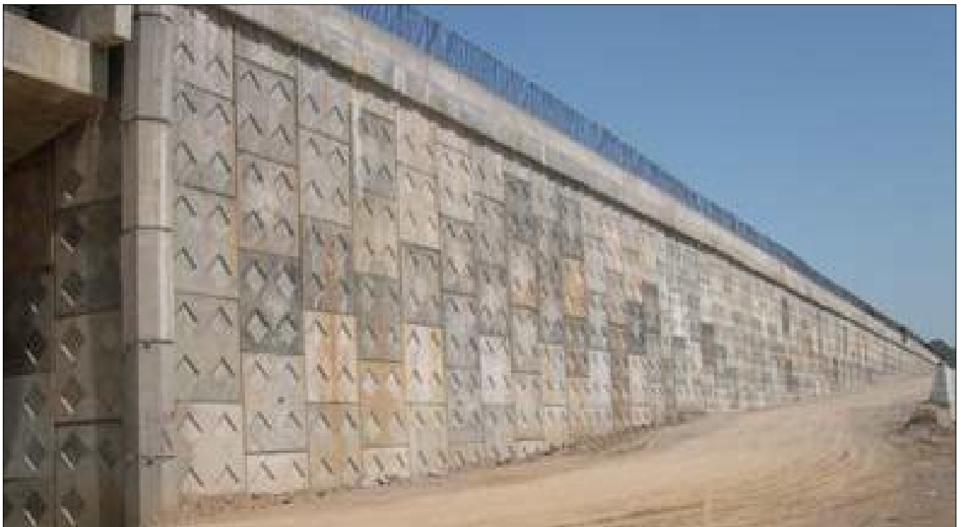
Photo 1 : Elevation view of RS Wall
