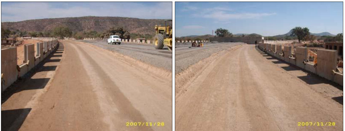
Photo 2 & 3: Erection of RS wall
