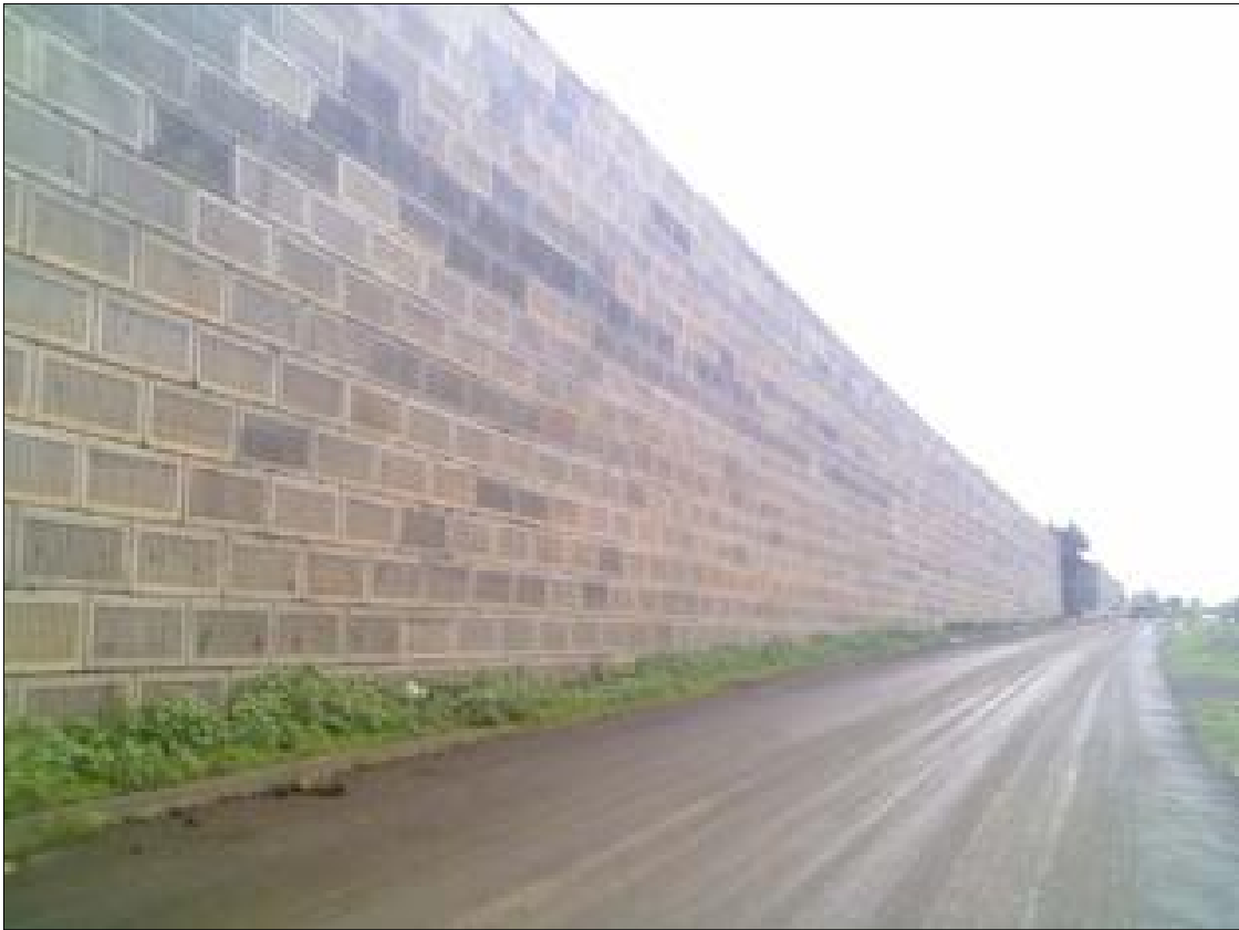
Elevation view of RS wall
