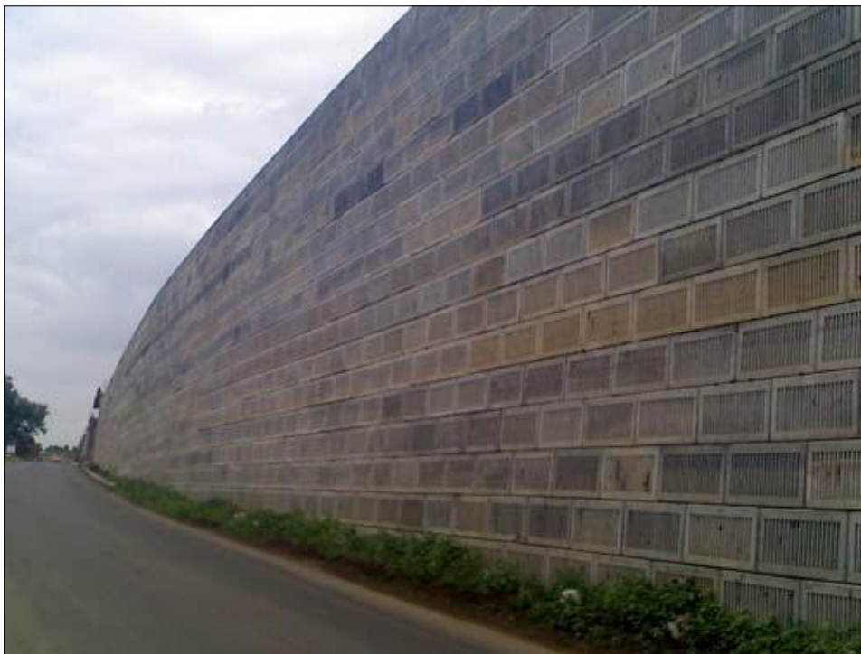
Photo 1 : Elevation view of Nagpur-Hyderabad Section
