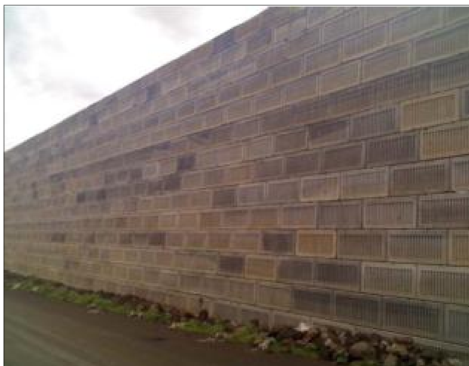
Elevation view of RS wall
