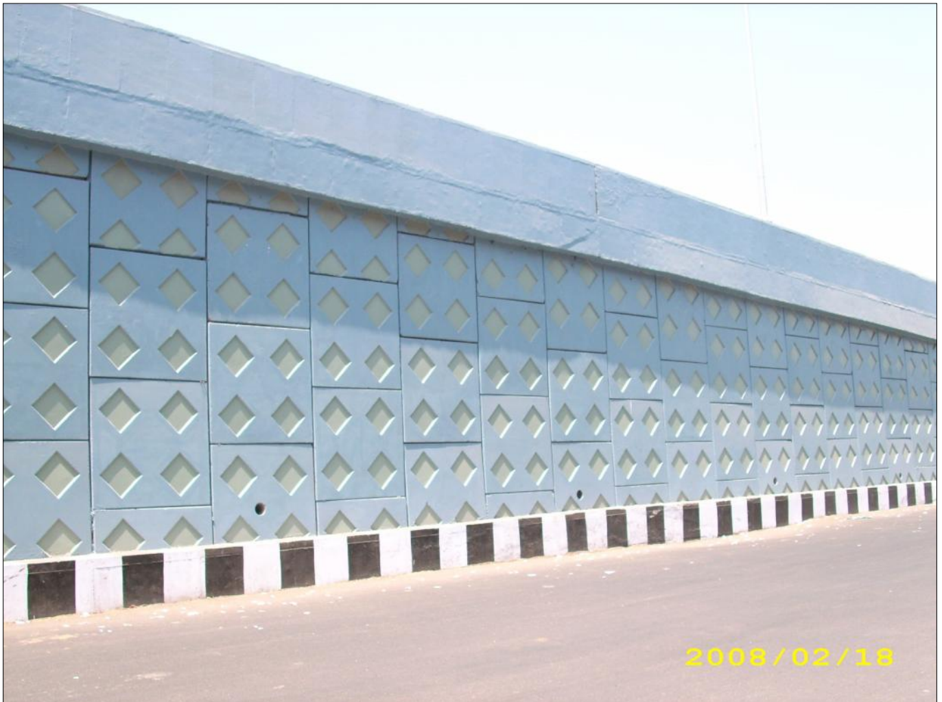
Elevation view of RS wall
