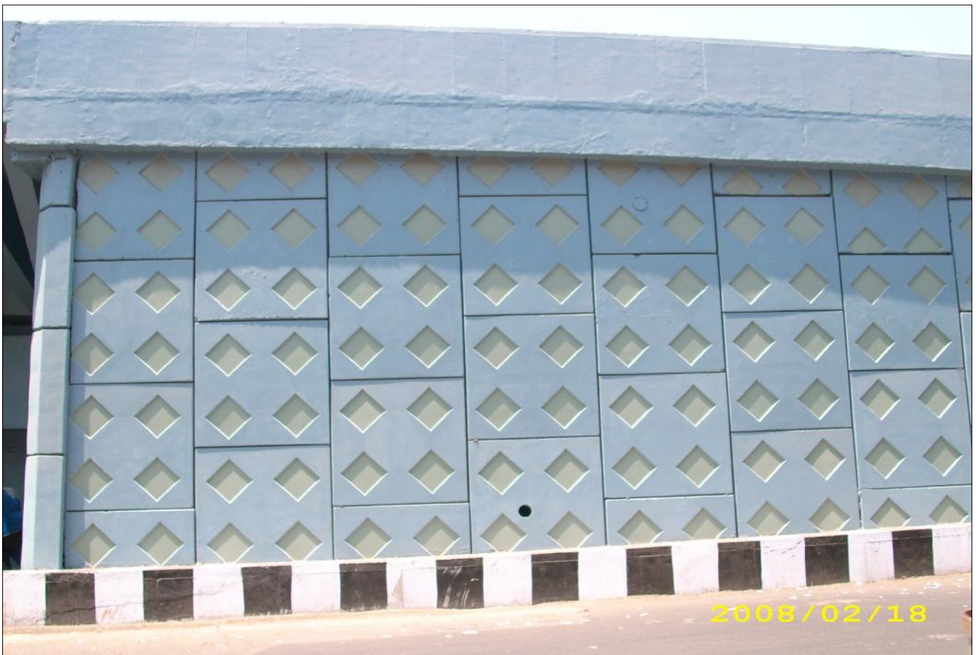
Elevation view of RS wall
