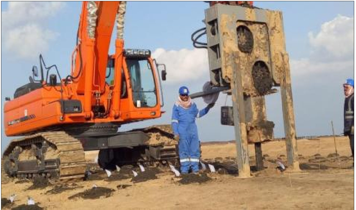
TechDrain PVD installation is in progress
