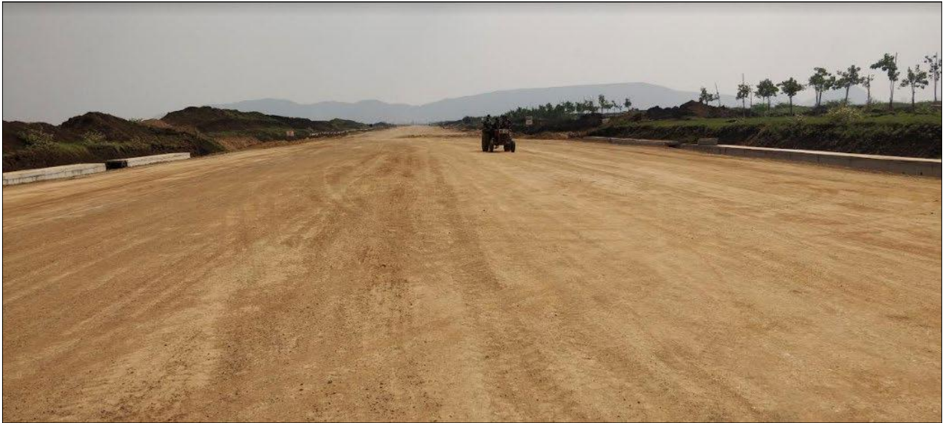
Prepared Subgrade before laying structural layers of the pavement
