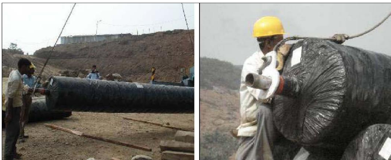
Handling of Geosynthetic Rolls
