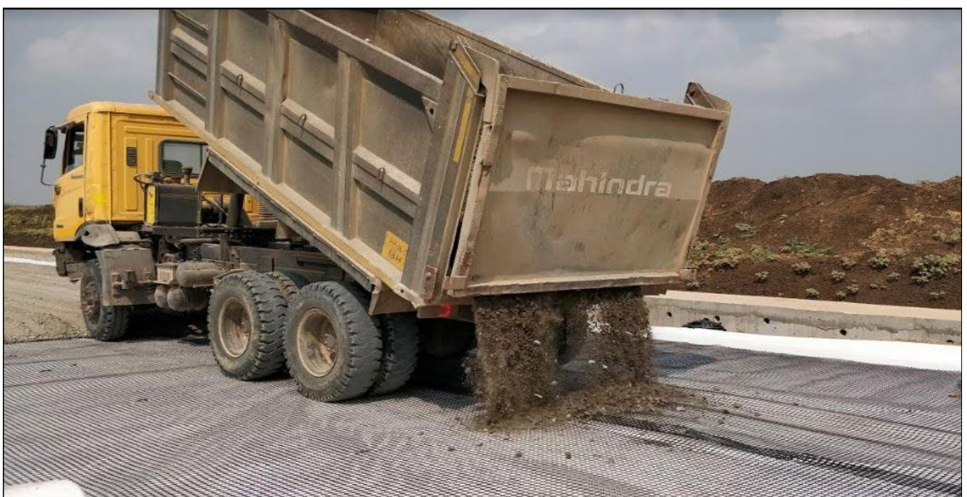
Dumping of GSB material on the geogrid + geotextile layer
