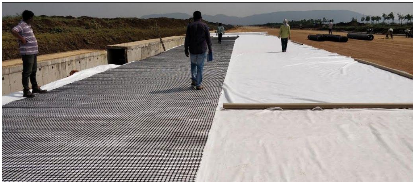
Unrolling of Geogrid & Geotextile and Inspection for any wrinkles
