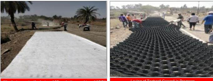
After laying geotextile, laying of 25mm bottom cushion of WMM
