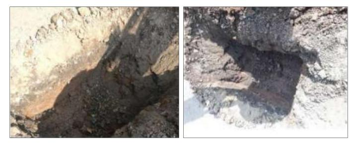
After site visit and detailed observation it is concluded that the softening of sub base layer can be the main reason of failure under heavy axle loading which was not anticipated. Conventional methods of pavement/soil improvement were already tried and which proved ineffective, so it is very important to offer solution considering the life of pavement; anticipated growth in traffic and cost.
