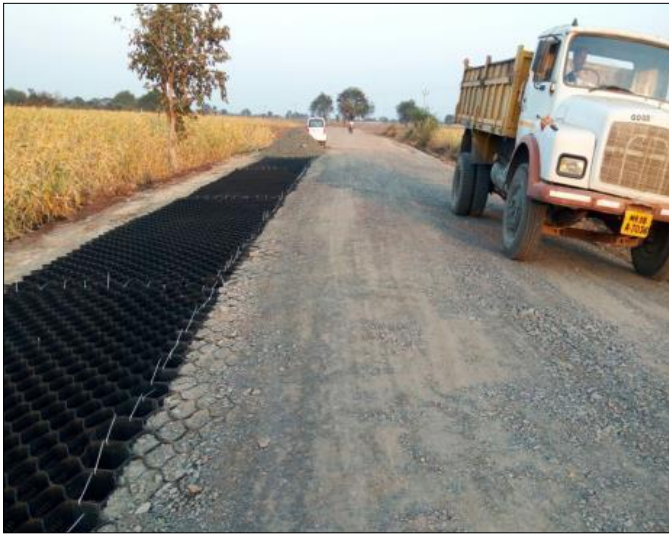
Laying of GSB in progress
