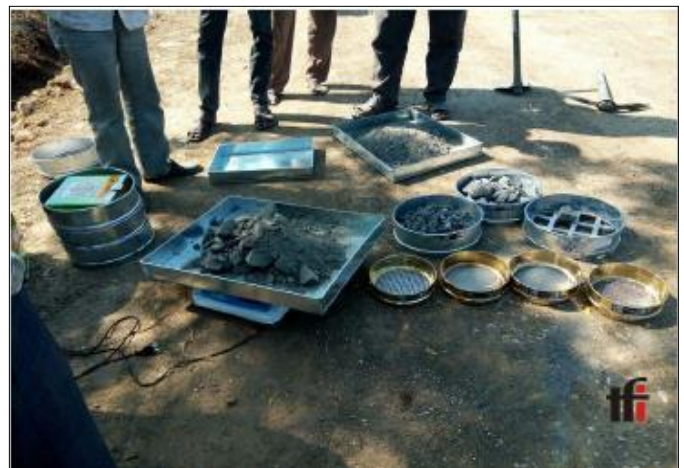
Gradation Test of GSB on site
