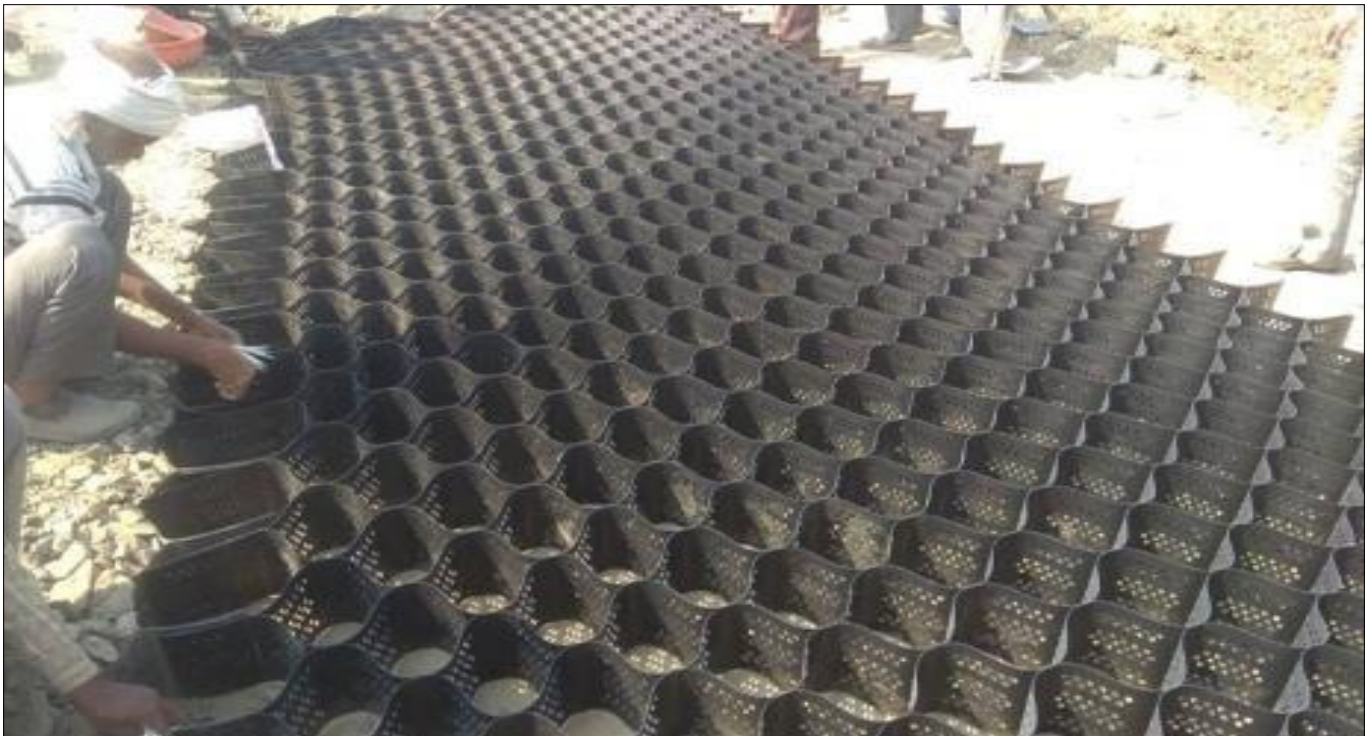
Techcell laying in progress
