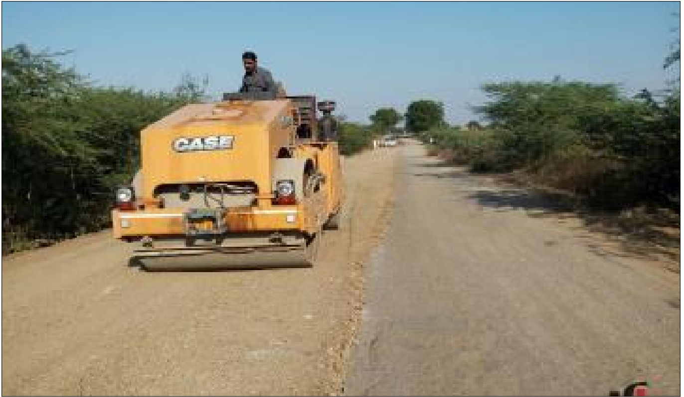
Sub-Grade compaction in progress
