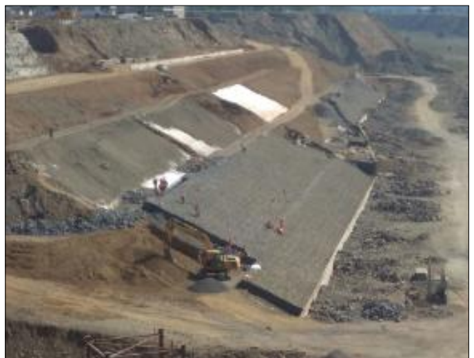
TechFab Metal Gabion Mattress laying in progress
