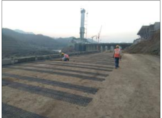
Geogrid Laying for RS Walls
