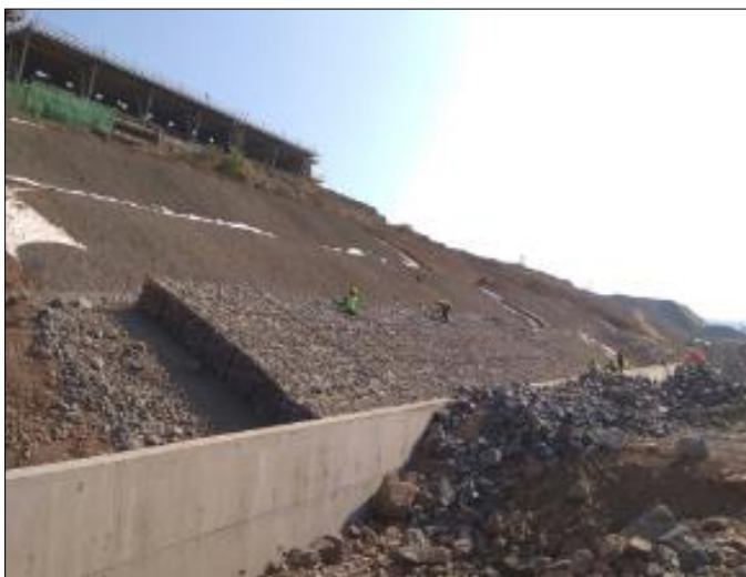
TechFab Metal Gabion Mattress laying in progress
