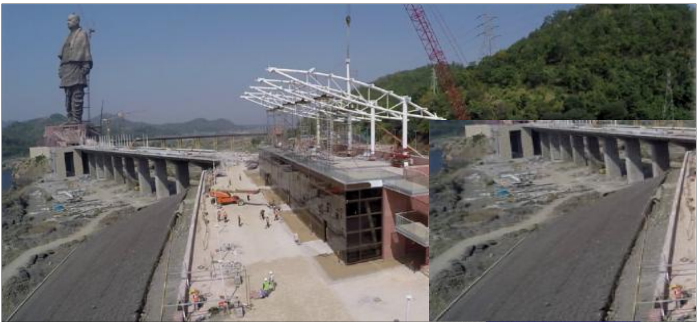
Panoramic View of TechFab products in the vicinity of Sardar Sarovar Dam
