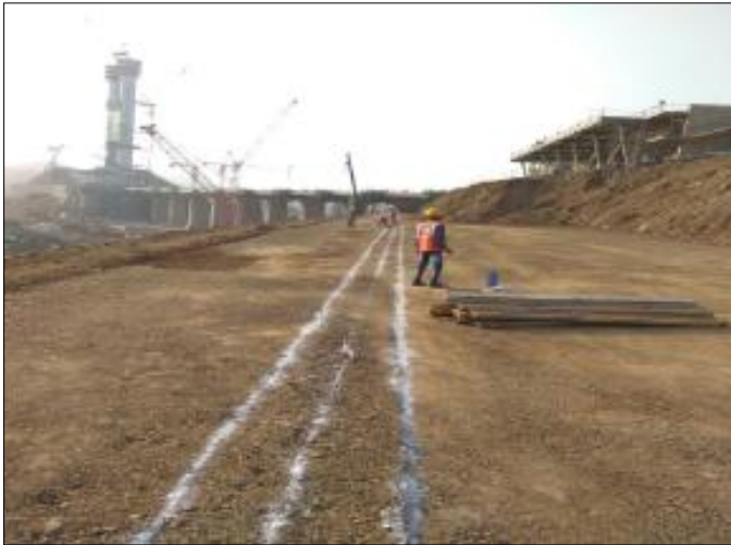
Marking in progress for RS Walls
