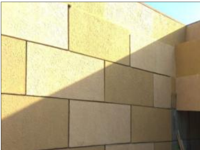
Finished view of RS Wall Panels
