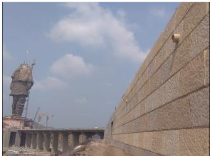
Finished view of RS Wall Panels
