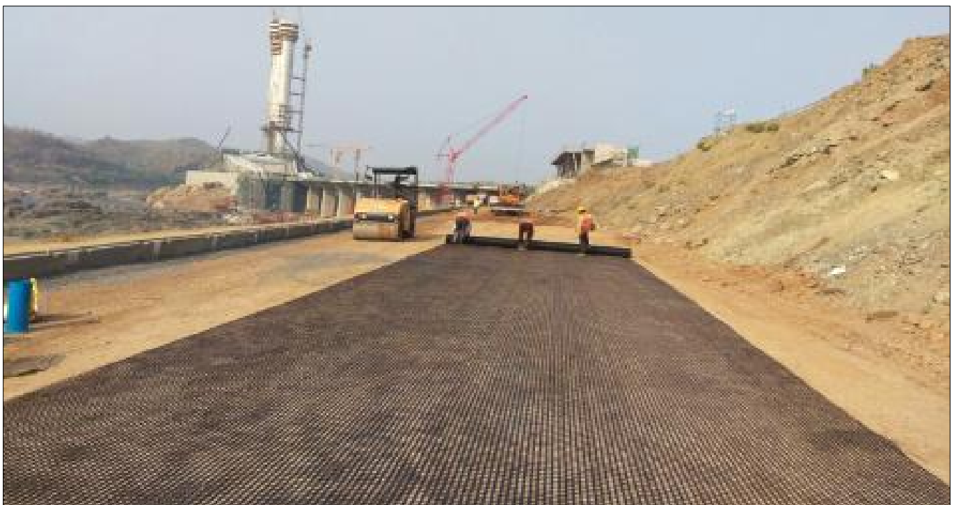
Laying of TechGrid Geogrid in Progress
