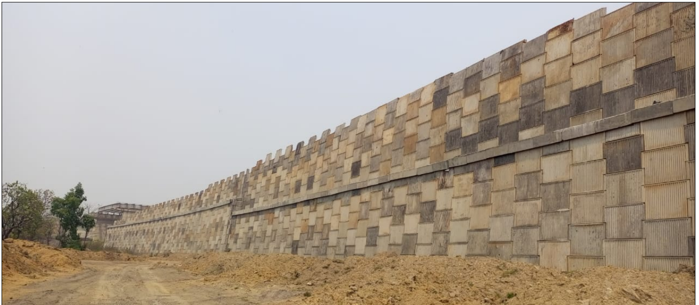
Photo 5 & 6 : Photographs of Completed Structure
