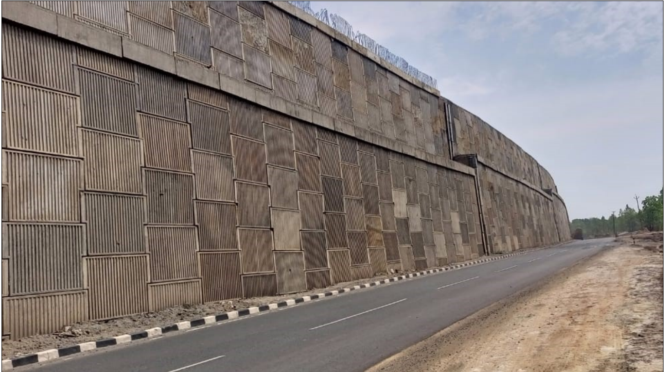
Photo 2 : Photograph of RSW on RHS side
