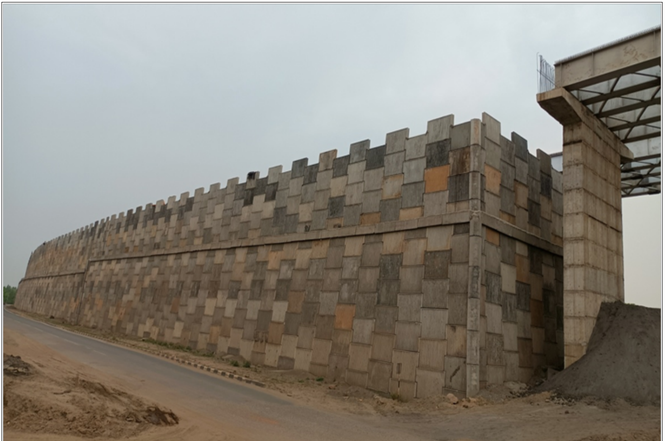
Photo 1 : Photograph of RSW on LHS side
