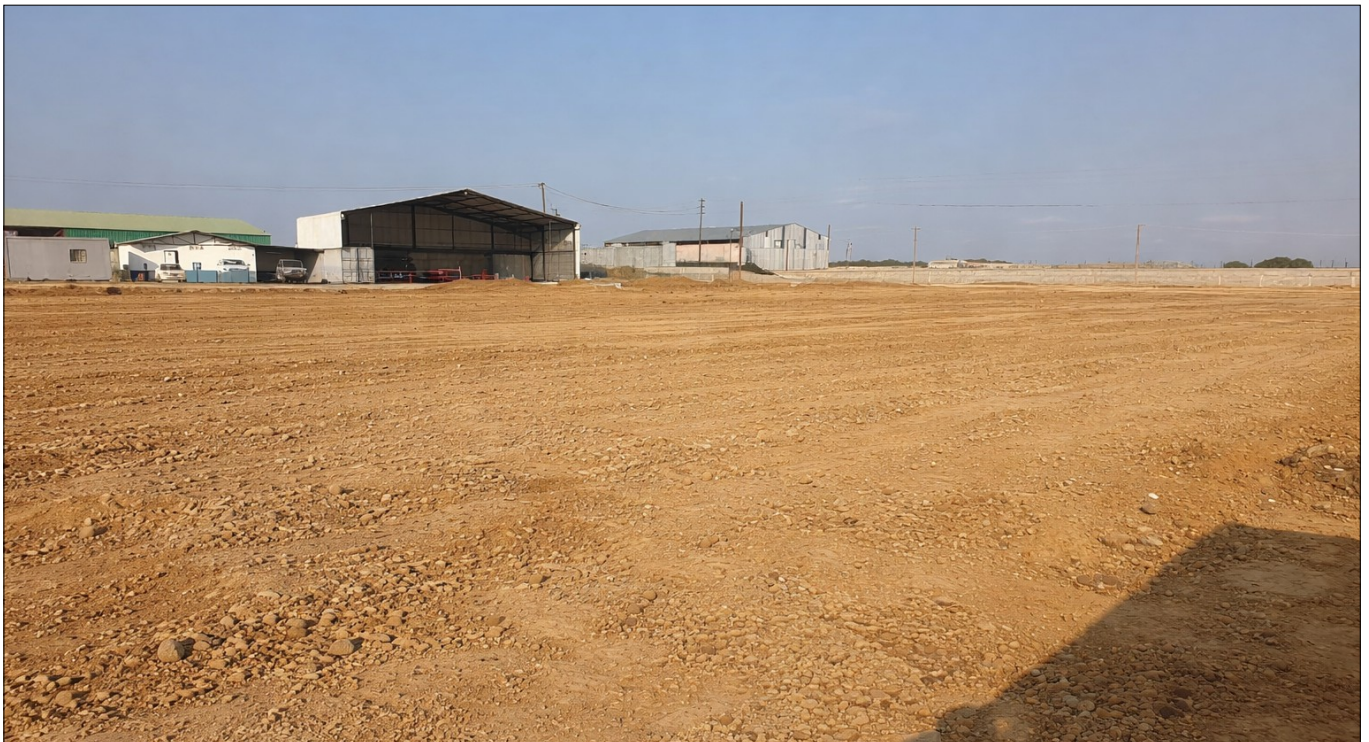
Photo 1: Prepared surface of container yard prior to installation of TGC Reinforced Nonwoven Geotextile
