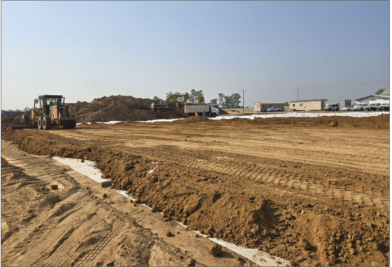
Photo 5 : Compaction of Soil Layer Over TGC Reinforced Nonwoven
