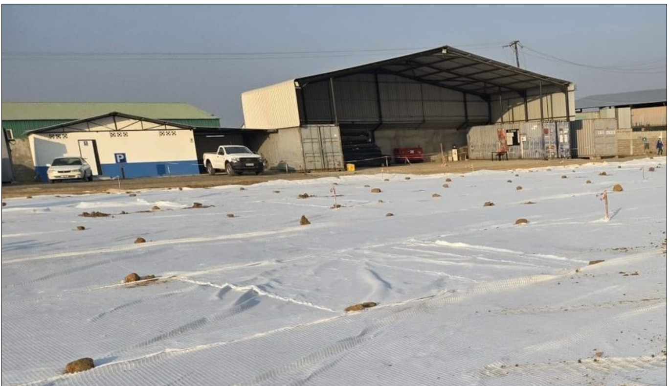
Photo 2 : installation of TGC Reinforced Nonwoven Geotextile
