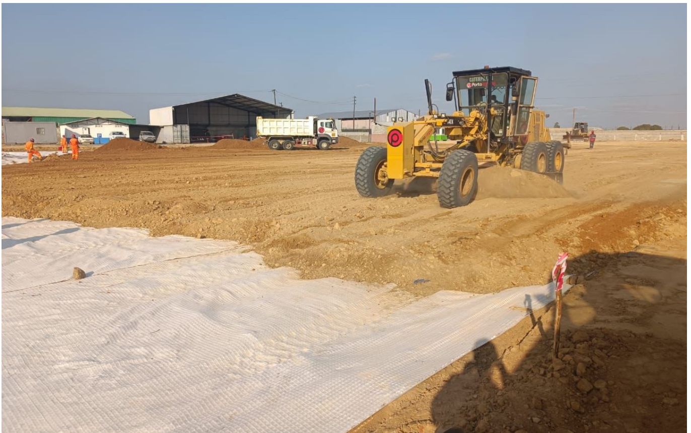
Photo 4 : Soil Spreading Over TGC Reinforced Nonwoven
