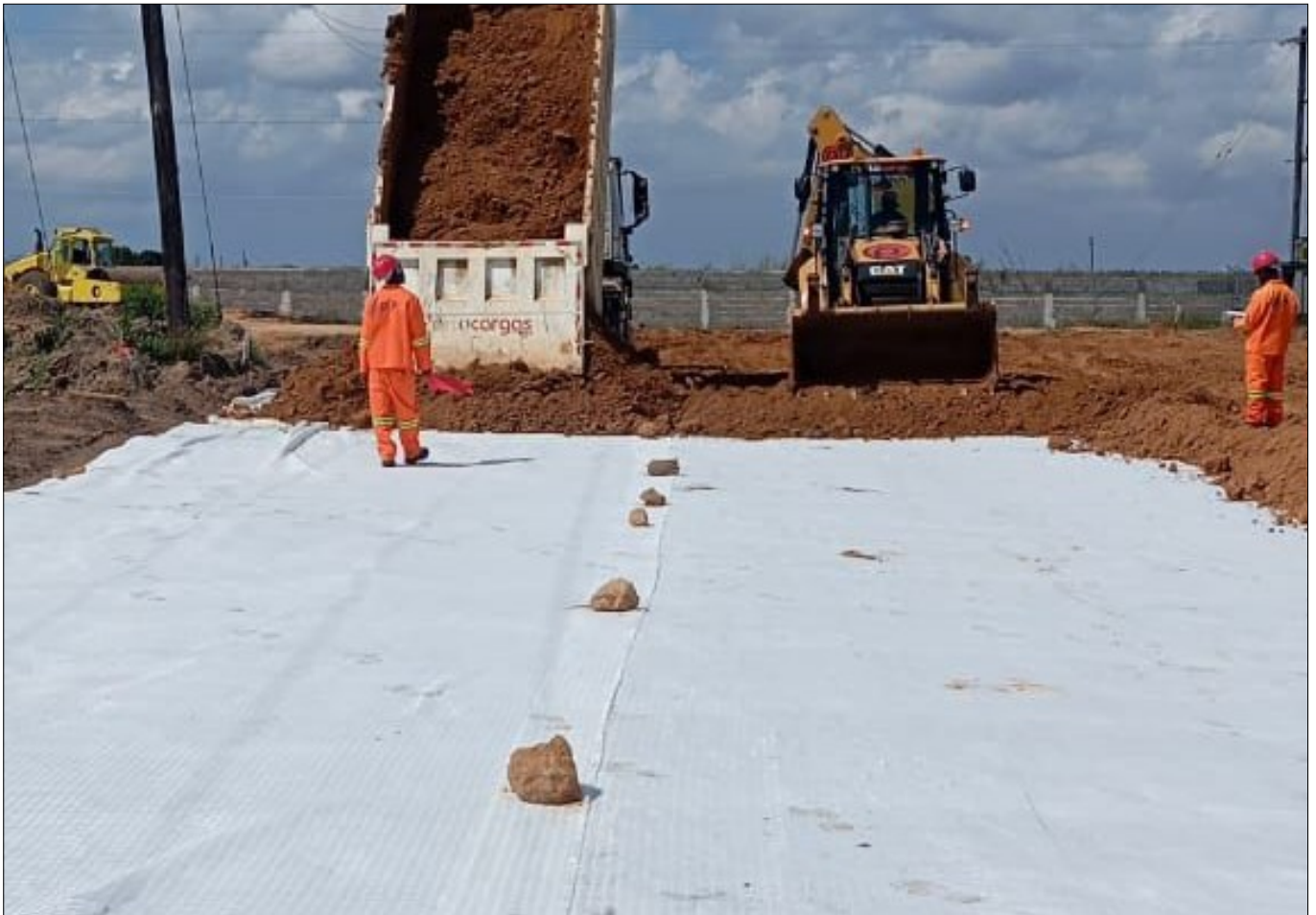
Photo 3 : Soil Placement Over TGC Reinforced Nonwoven Geotextile
