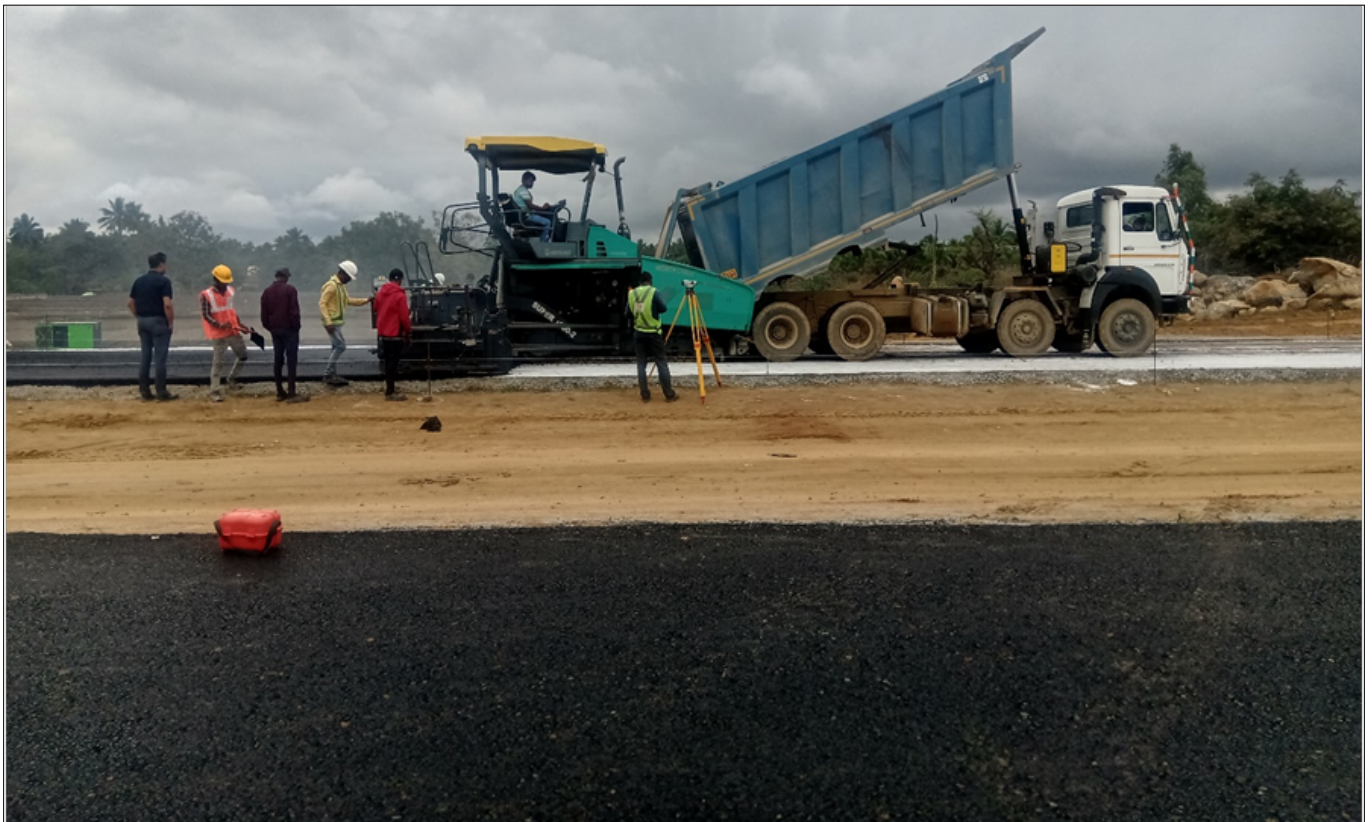
Photo 4 : Laying of DBM layer
