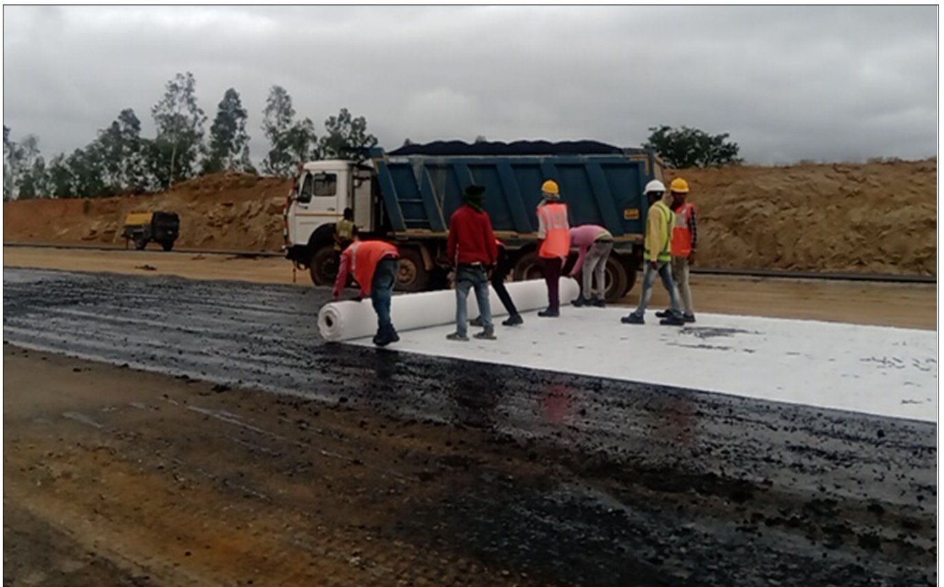
Photo 2 : Laying of Paving Fabric on Tack Coat
