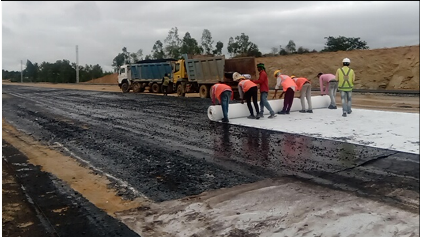
Photo 3 : Laying of Paving Fabric
