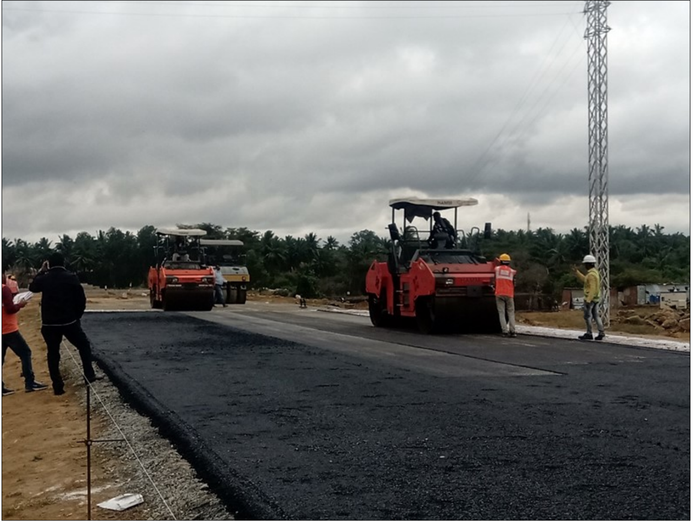
Photo 5 : Compaction of DBM layer
