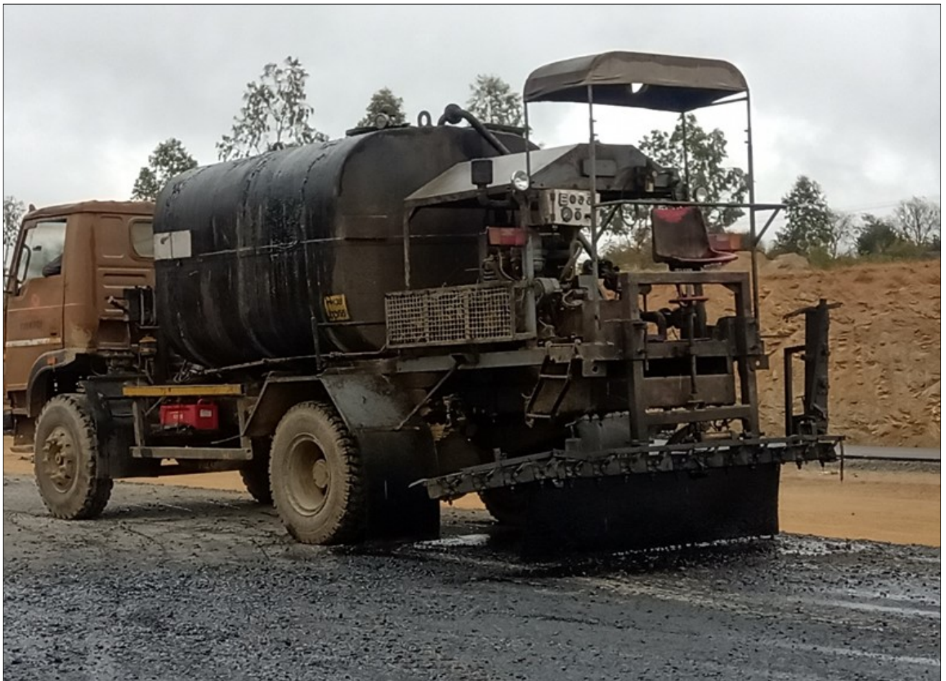
Photo 1 : Laying OF Tack Coat Before Overlaying of Paving Fabric
