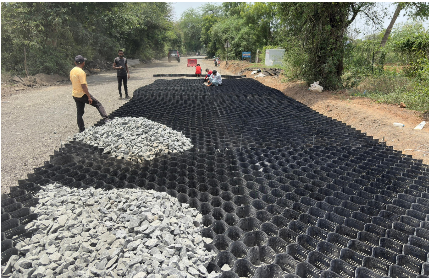
Photo 4 : Filling of GSB Material over TechCell Geocell
