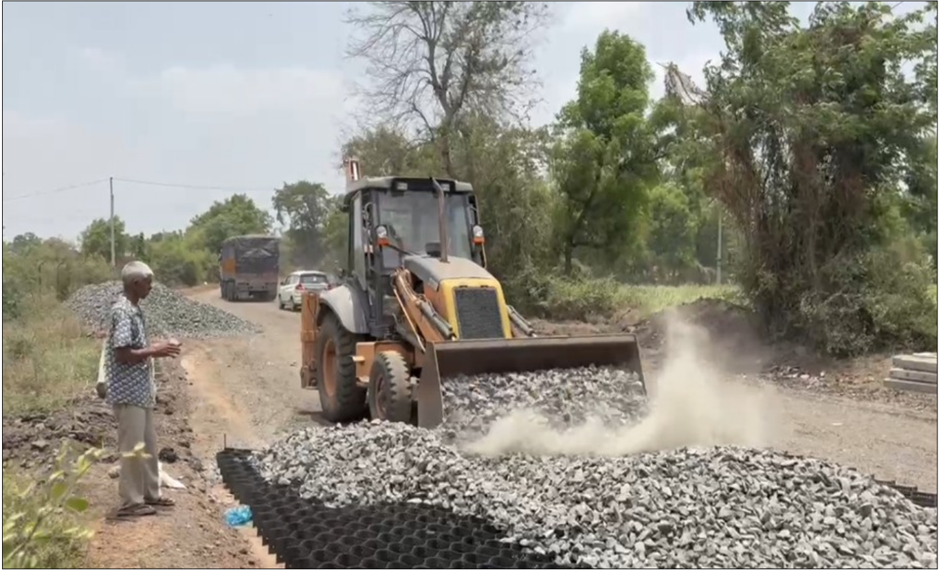
Photo 5 : Filling of GSB Material over TechCell Geocell
