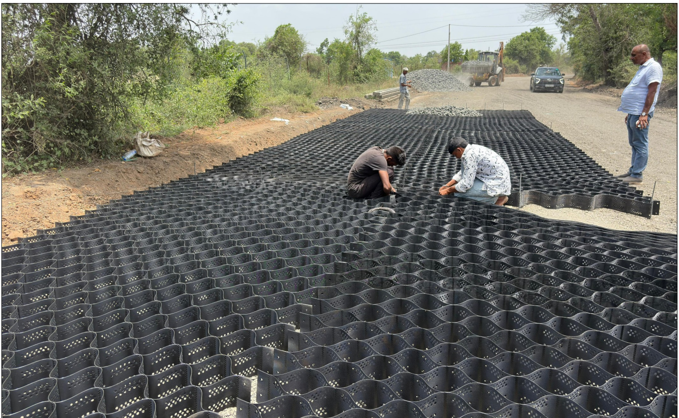
Photo 3 : Joining the Geocell panels with cable ties
