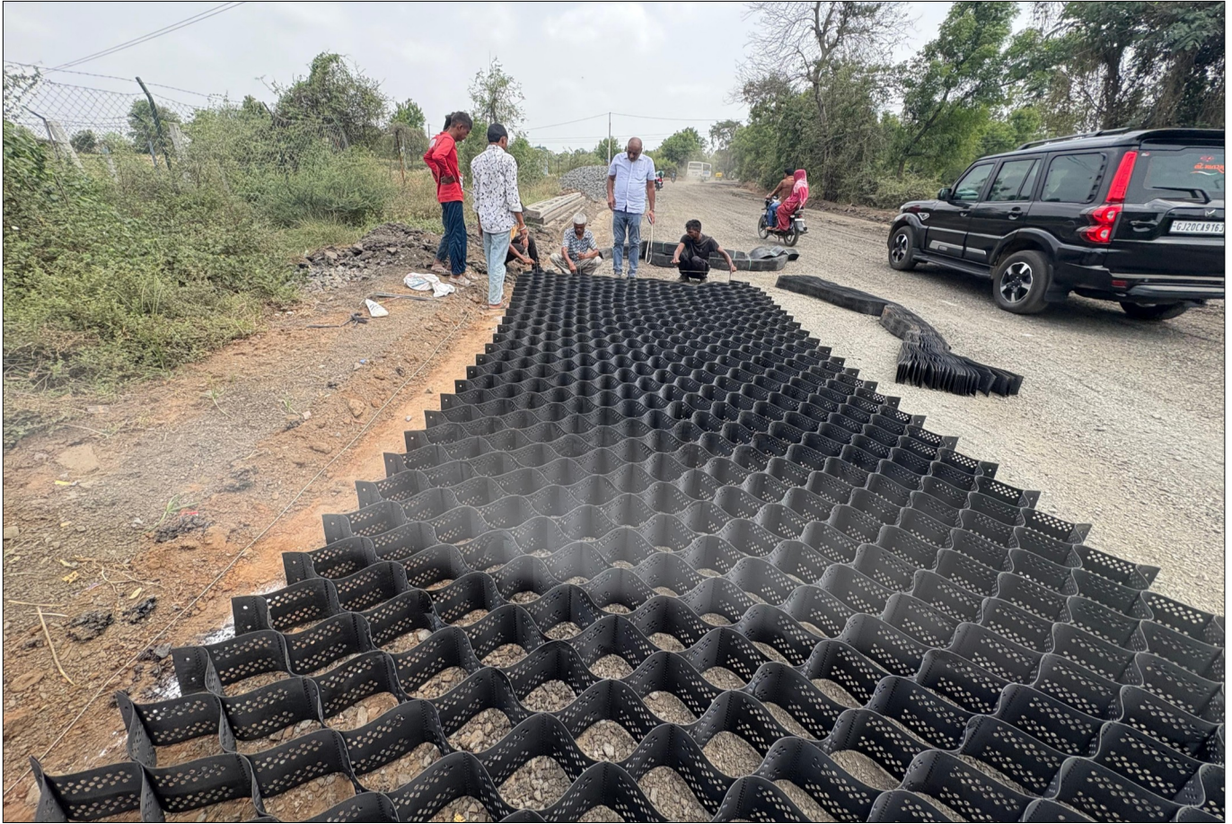
Photo 2 : Installation of TechCell Geocell
