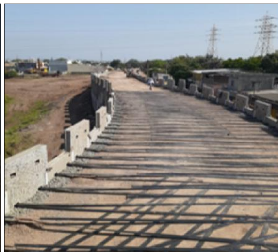
Installation of top layer TechStrap Polymeric Strip
