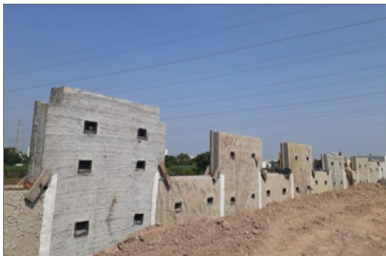
Erection of RCC Facia Panel in Progress
