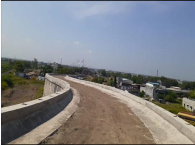
Coping beam installation completed
