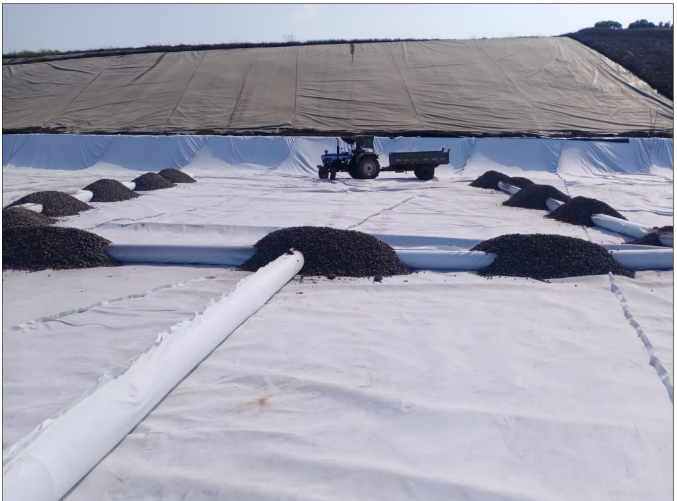
Photo 3 : Laying of Techgeo Nonwoven Geotextile
