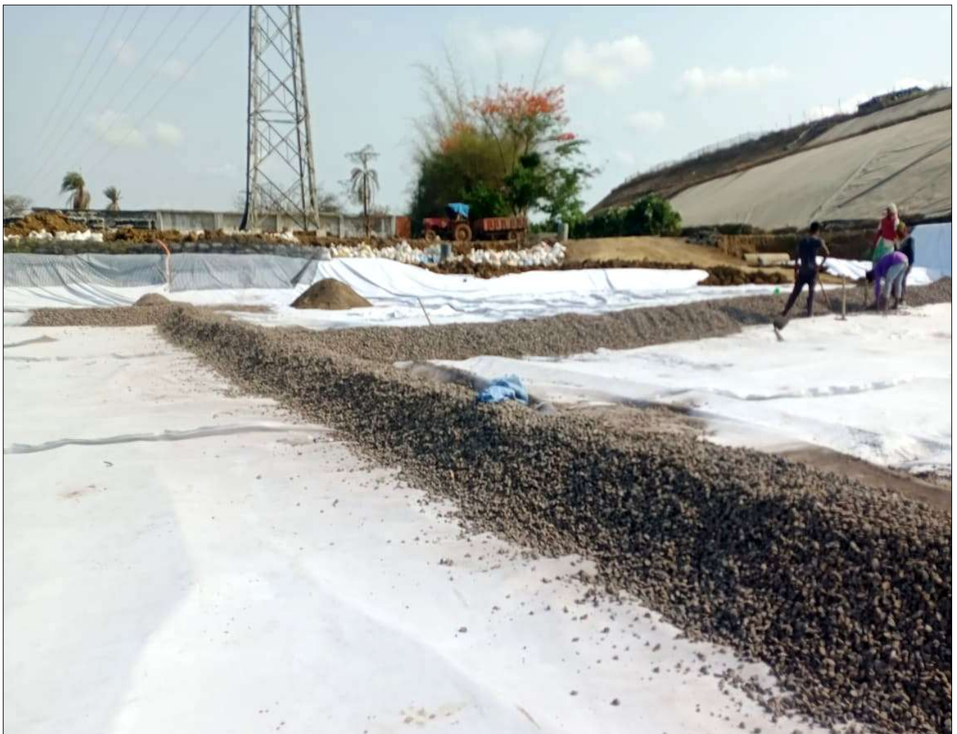
Photo 6 : Laying of Drainage Composite
