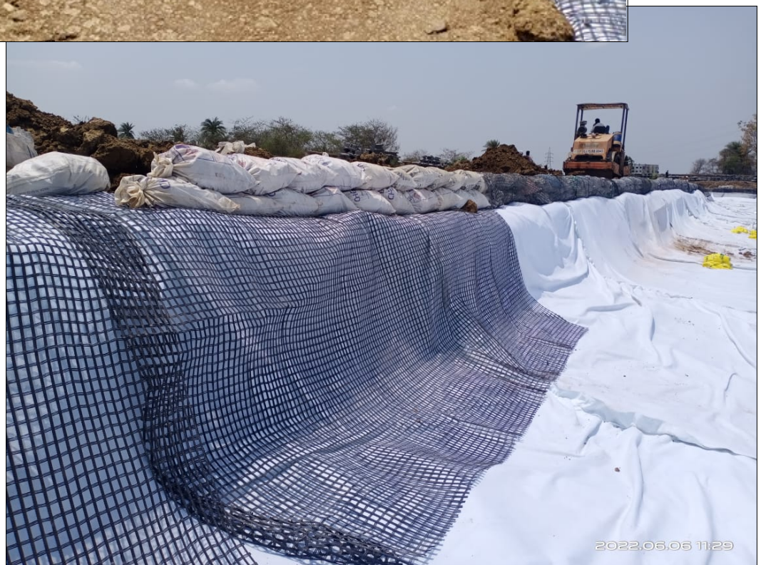
Photo 4 & 5 : Construction of Reinforced Earthen Wall Using TechGrid Uniaxial Geogrid
