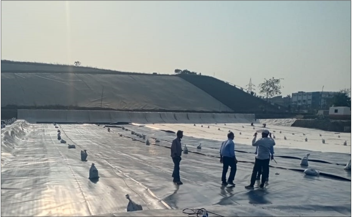
Photo 7 : After Construction Photograph
