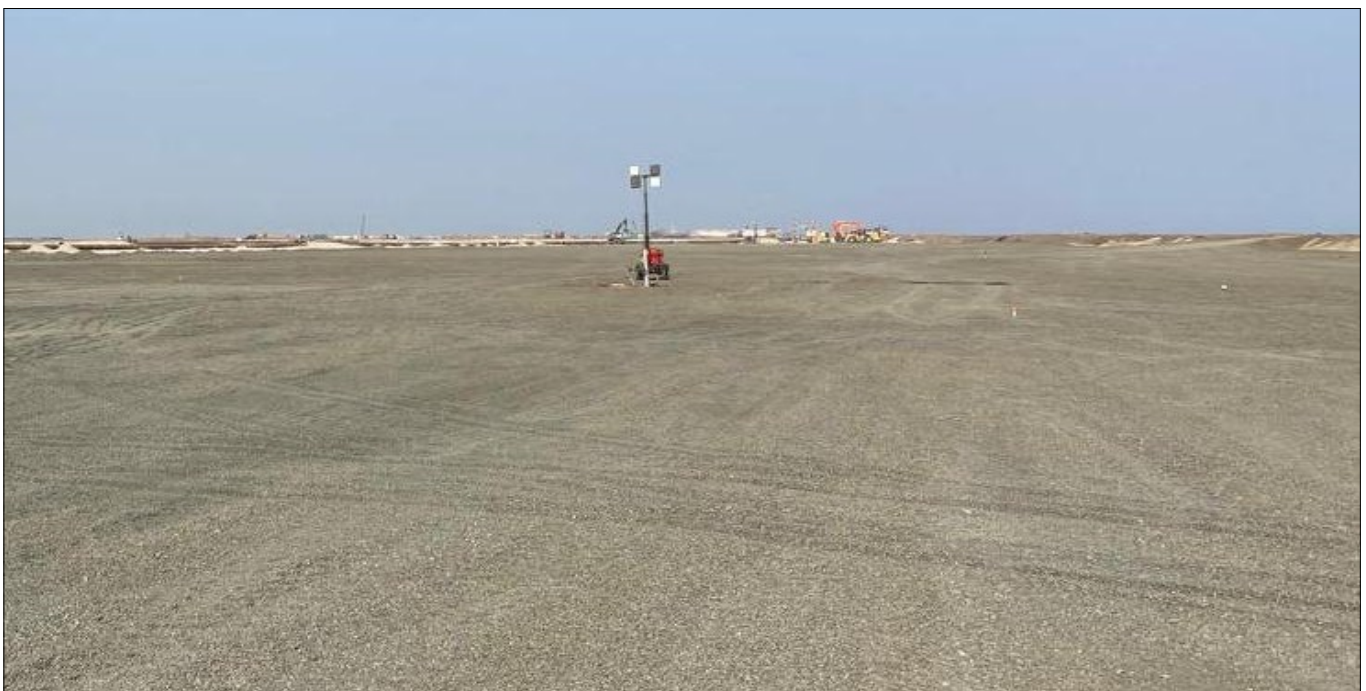
Photo 1: Site Prepared Prior to Protection Works
