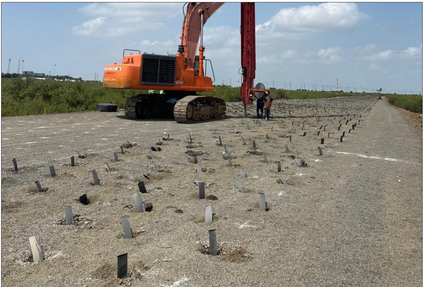
Photo 3 & 4 : TechDrain PVD Installation in Progress
