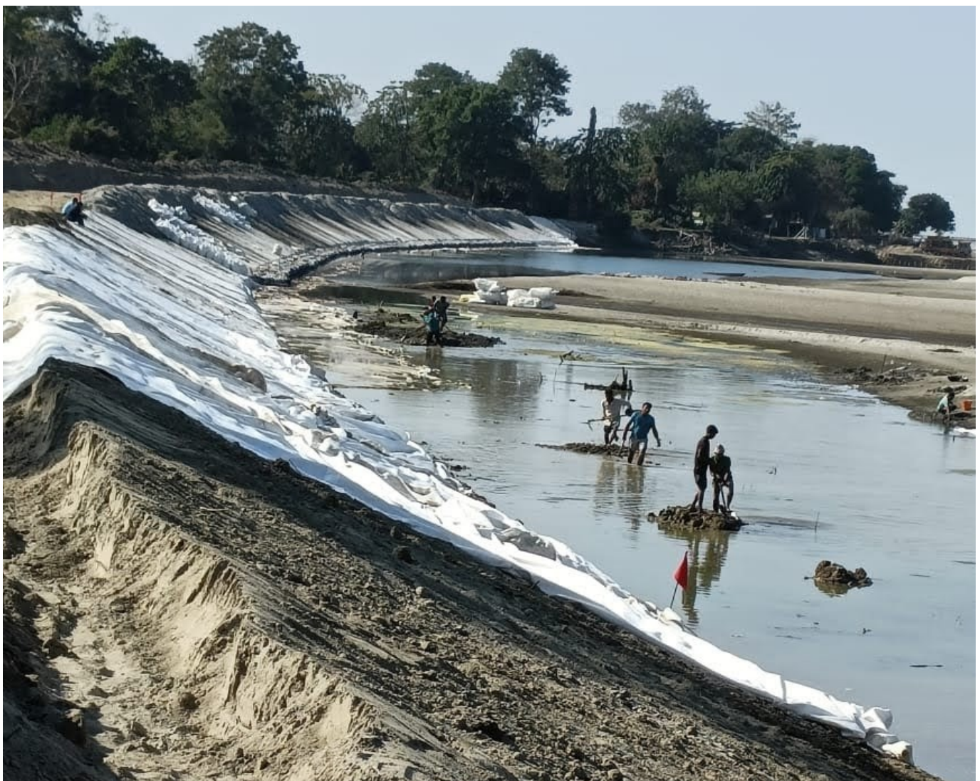
Photo 2 : Laying of TechGeo Nonwoven Geotextile on Dressed Slope
