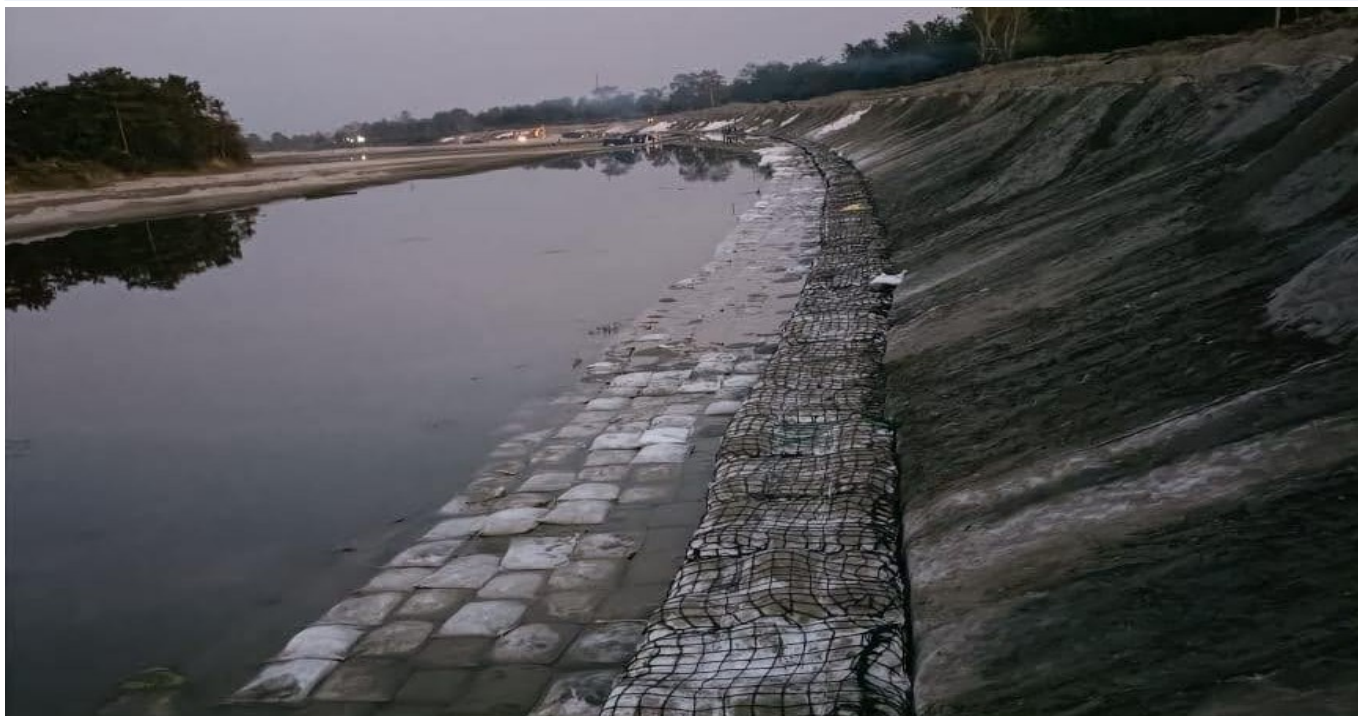
Photo 3 : installation of Geotextile Bags on River bed (For Launching Apron)
