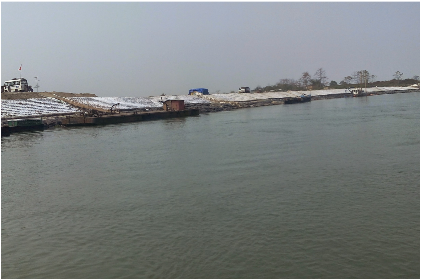
Photo 4 & 5 : Laying of Geotextile Bags on Slope
