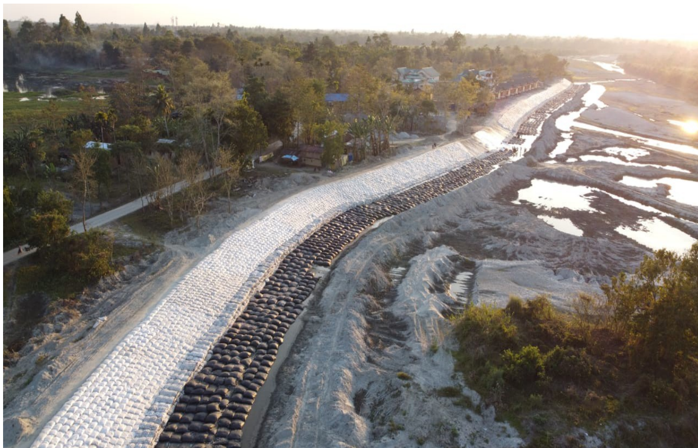
Photo 6 : After Completion Photograph
