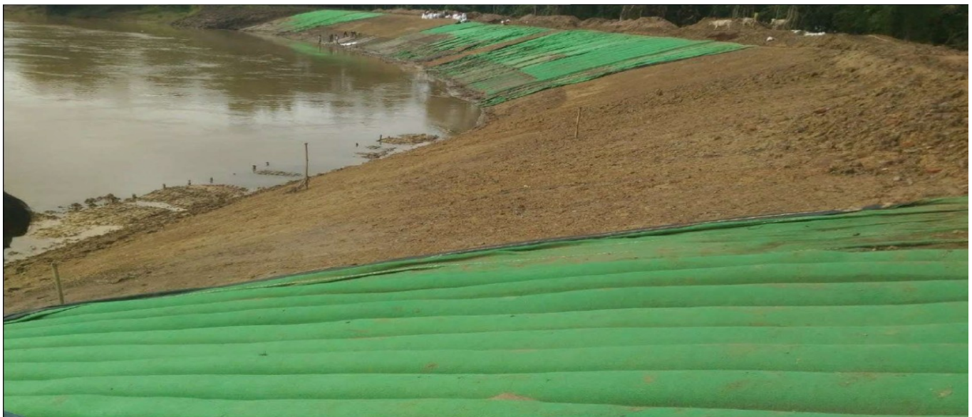
Photo 2 : Laying of Tech GeoMattress on Dressed Slope
