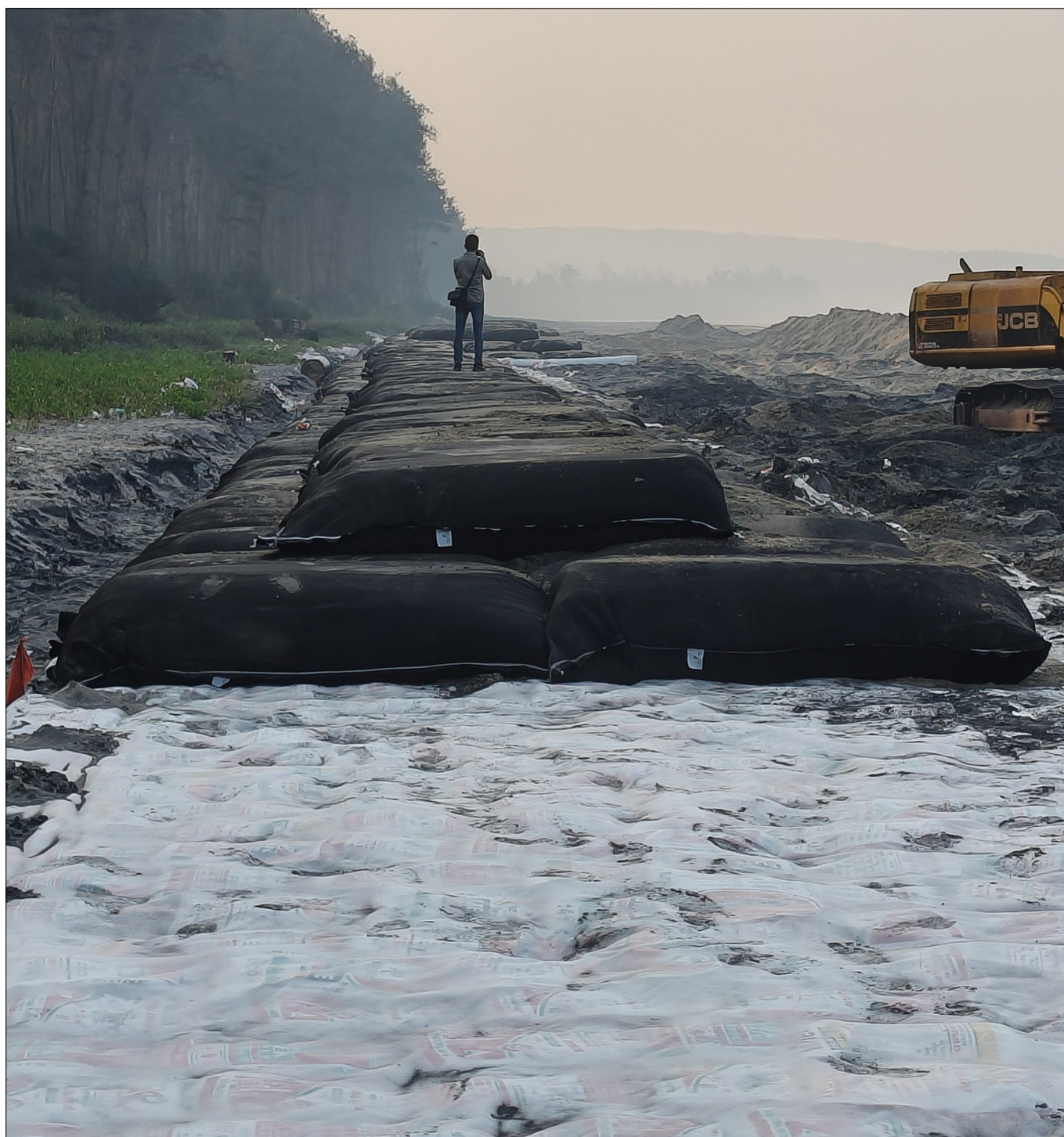
Photo 2 : Installation of Geobags
