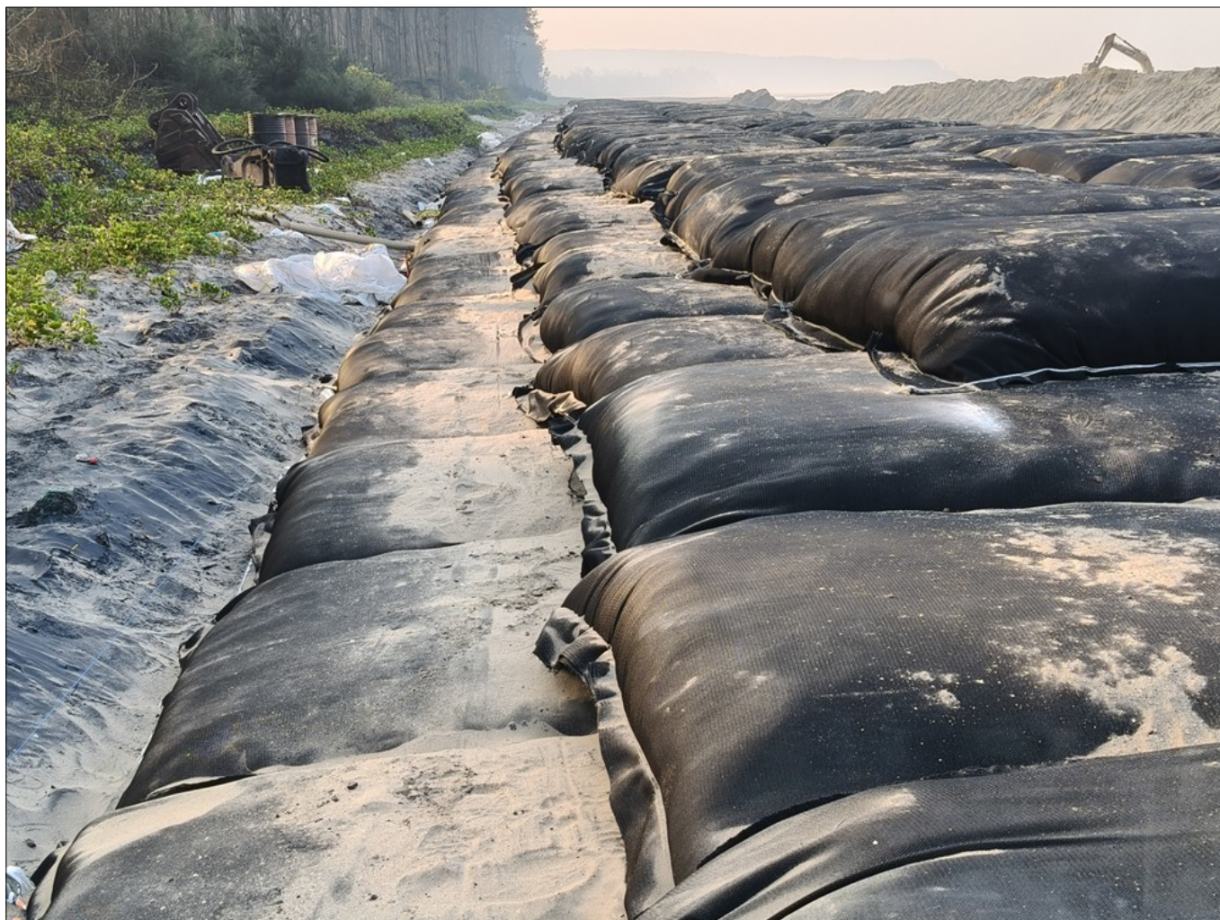
Photo 5 : Completed Geobag Works for Shore Protection
