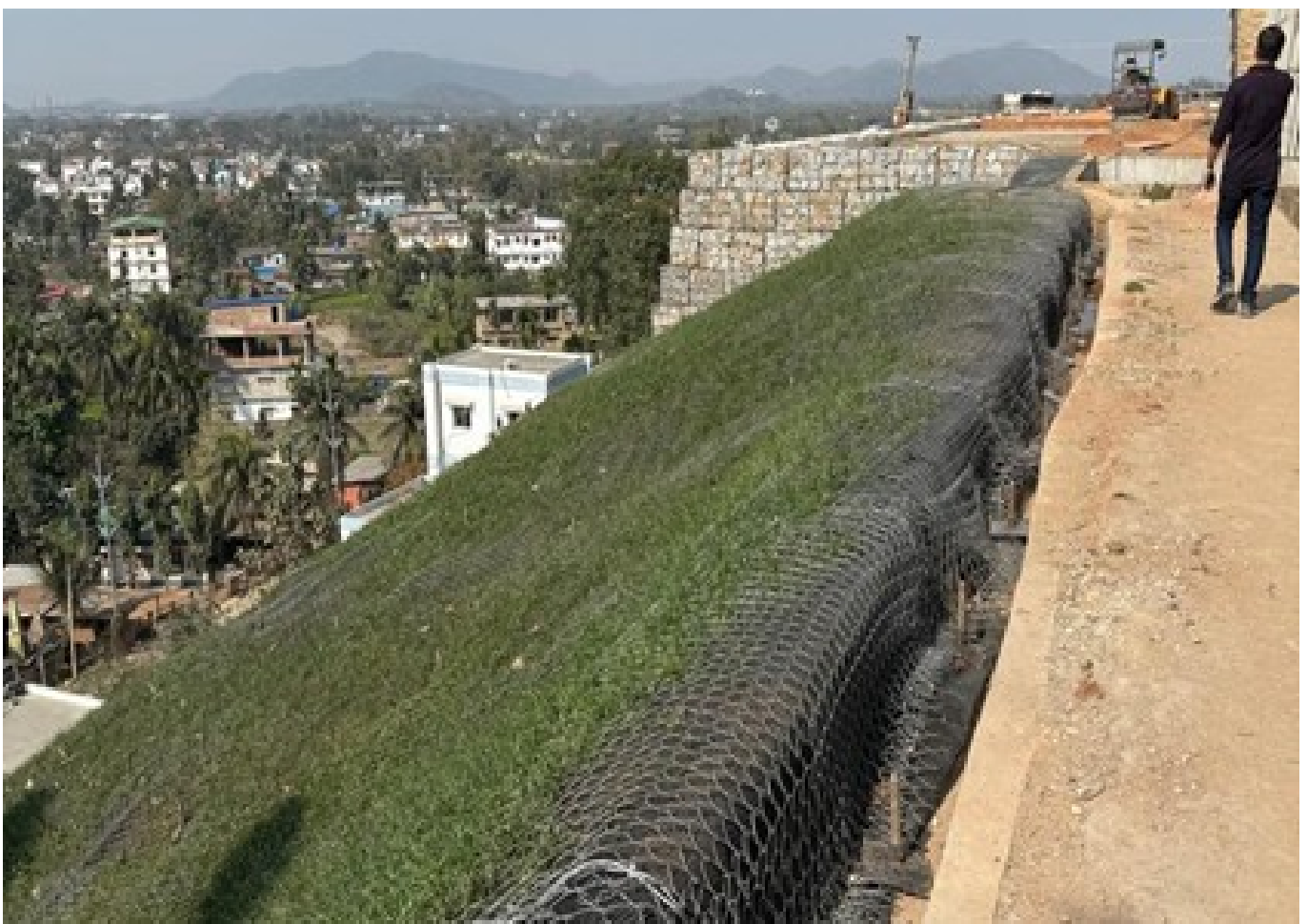
Photo 3 & 4 : Completed Installation of Slope Mitigation measures safeguarding the slope and adjoining infrastructure
