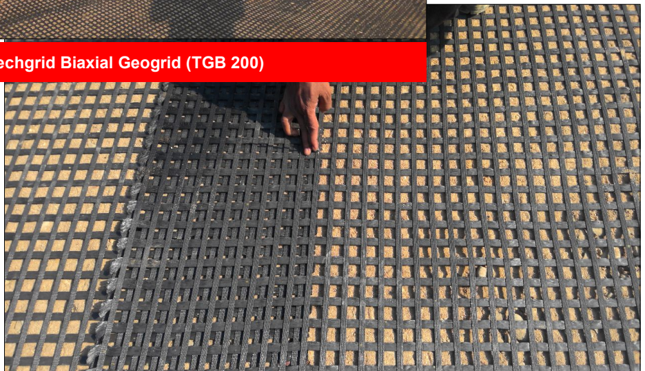
Photo 3 : Geogrid overlaps at the side edges
