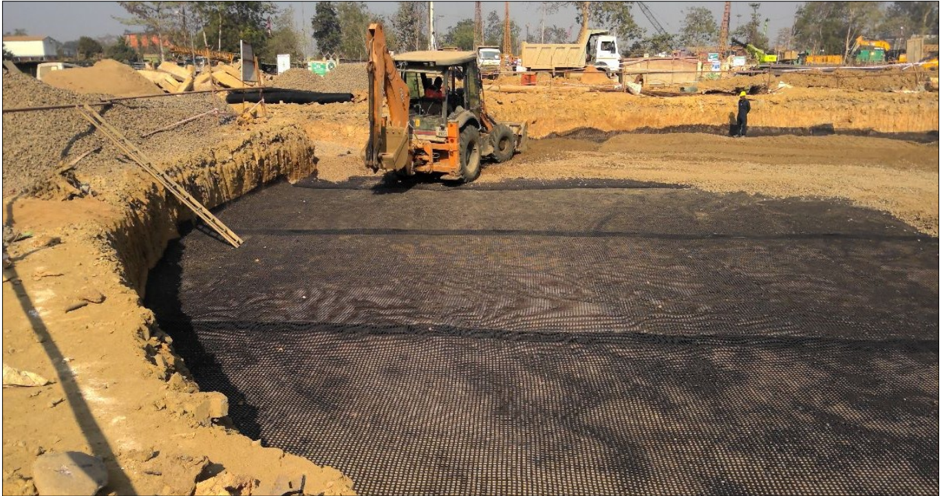
Photo 6 : Spreading of Fill Material
