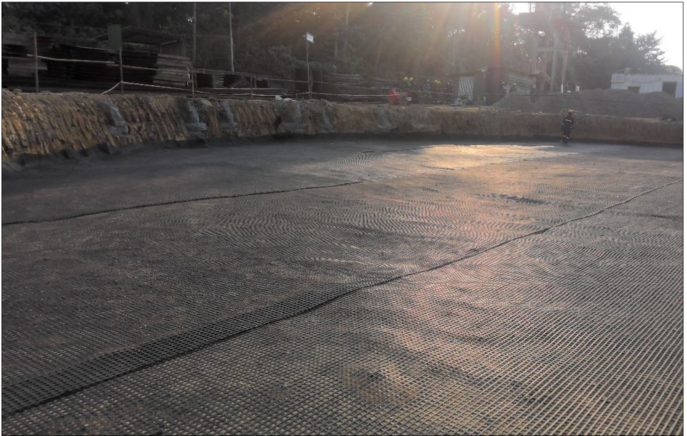
Photo 4 : After laying of geogrid layer
