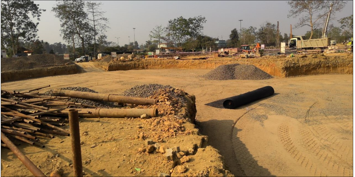
Photo 1 : Prepared Surface for Laying Geogrid & Rolls of Geogrids are ready to be laid
