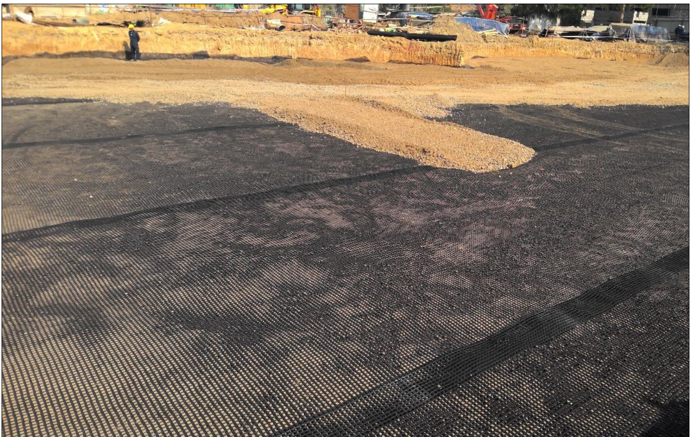
Photo 5 : Spreading of Fill material over geogrid
