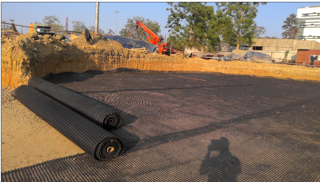
Photo 2 : Laying of Techgrid Biaxial Geogrid (TGB 200)
