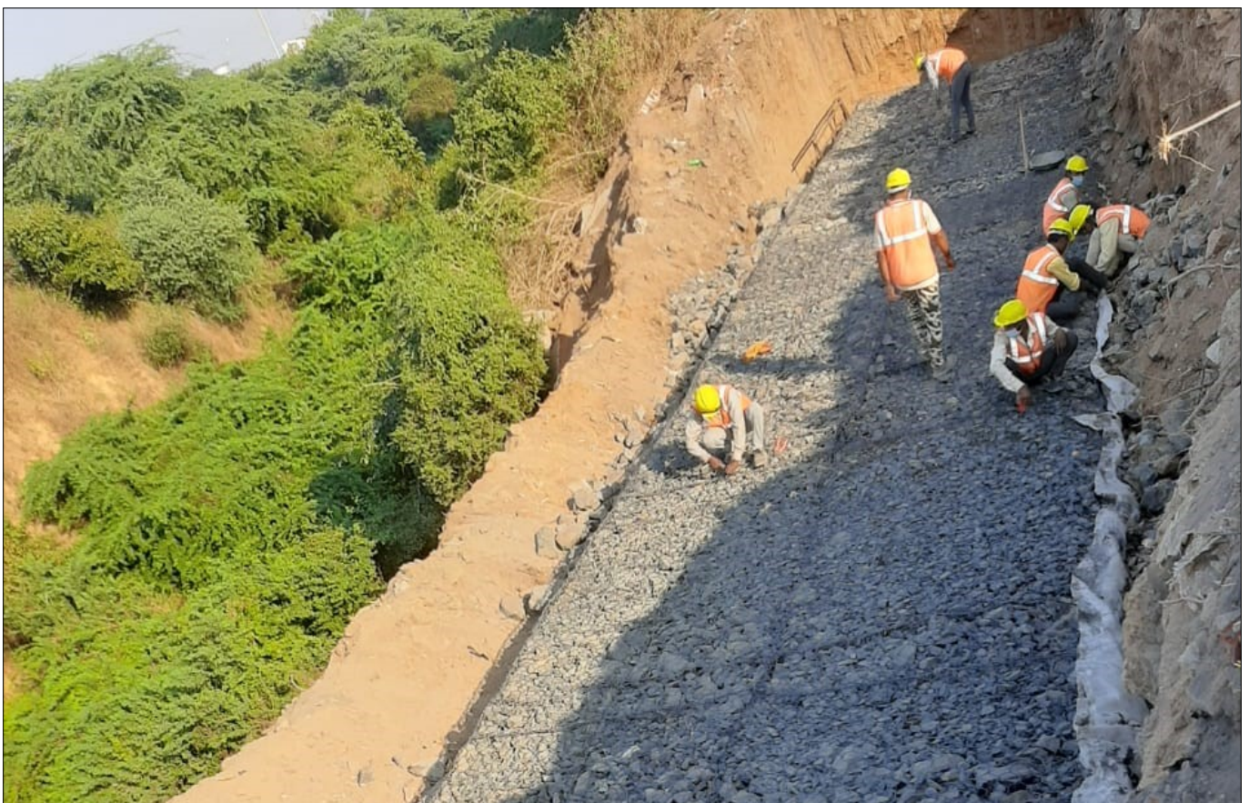
Photo 4 : Installation of Gabion Mattress at the Toe of the Wall to prevent Scouring
