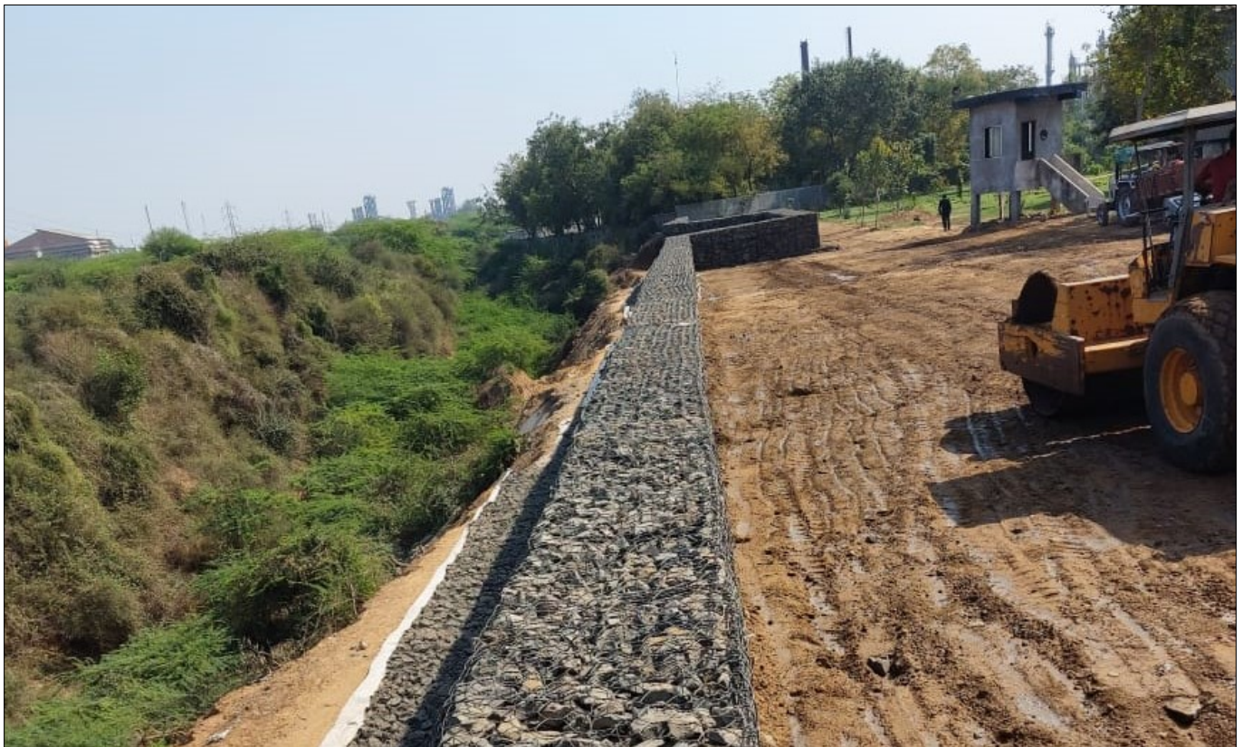
Photo 1 : During Construction Photograph
