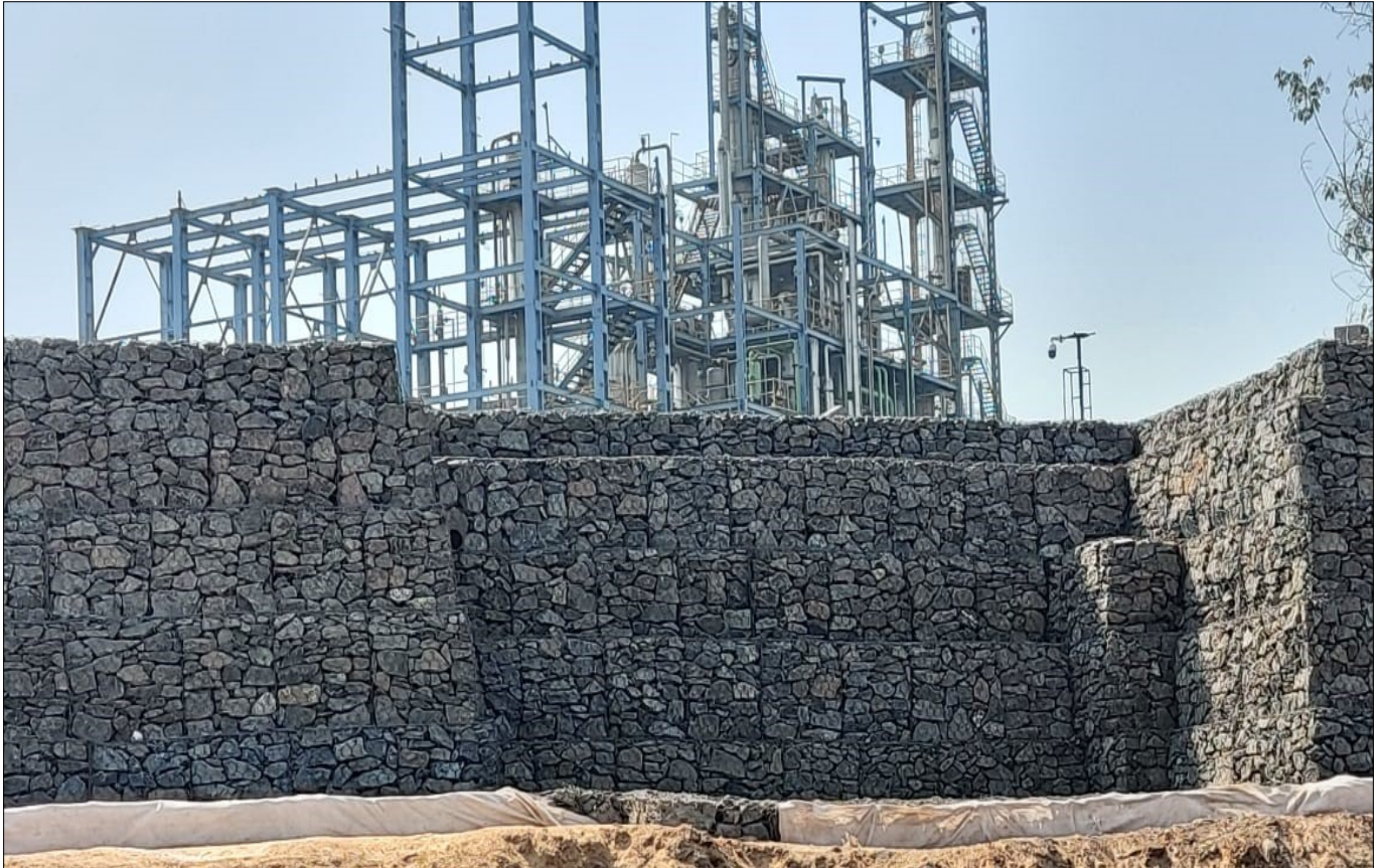
Photo 3 : Installation of Gabion Wall
