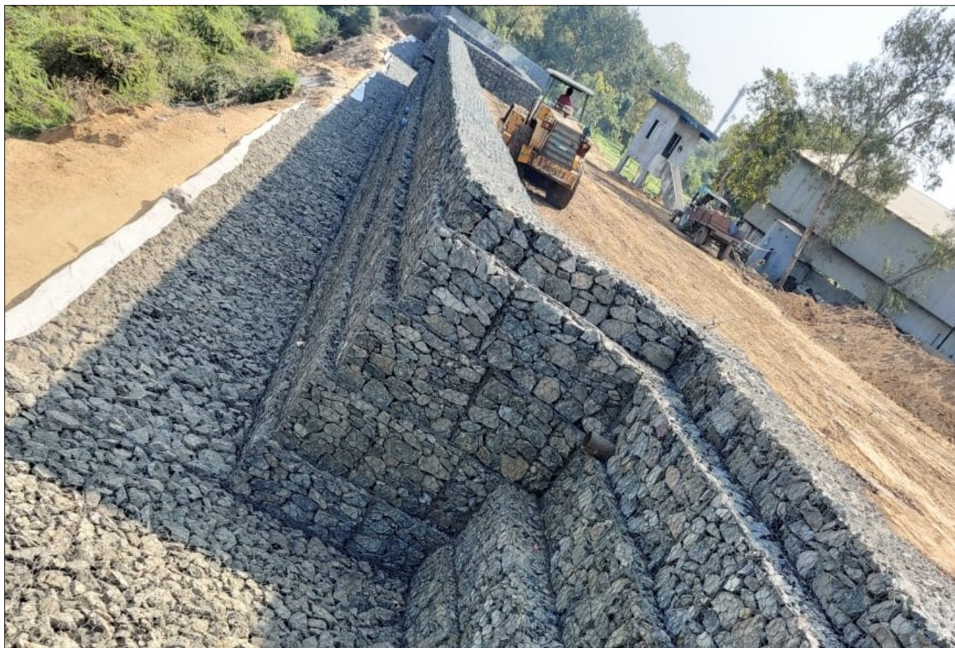
Photo 2 : During Construction Photograph
