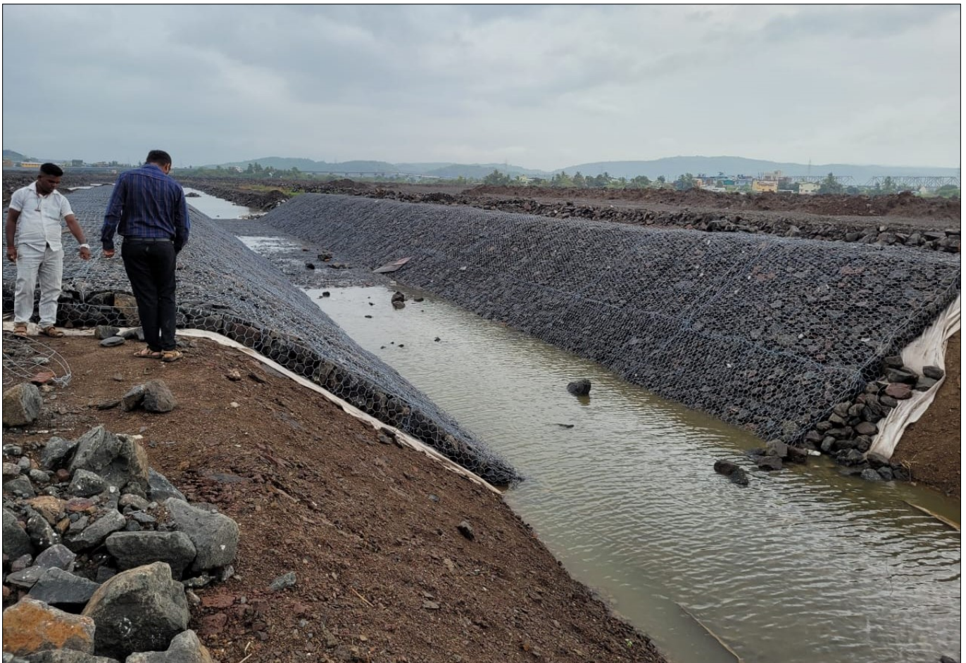
Photo 3 & 4 : During Construction Photographs
