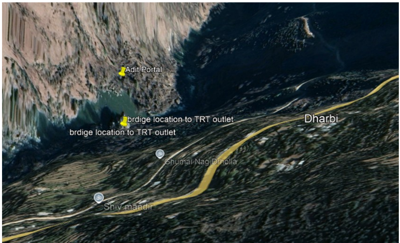
Photo 1 : Aerial View of TRT Adit Portal and Proposed Bridge Location
