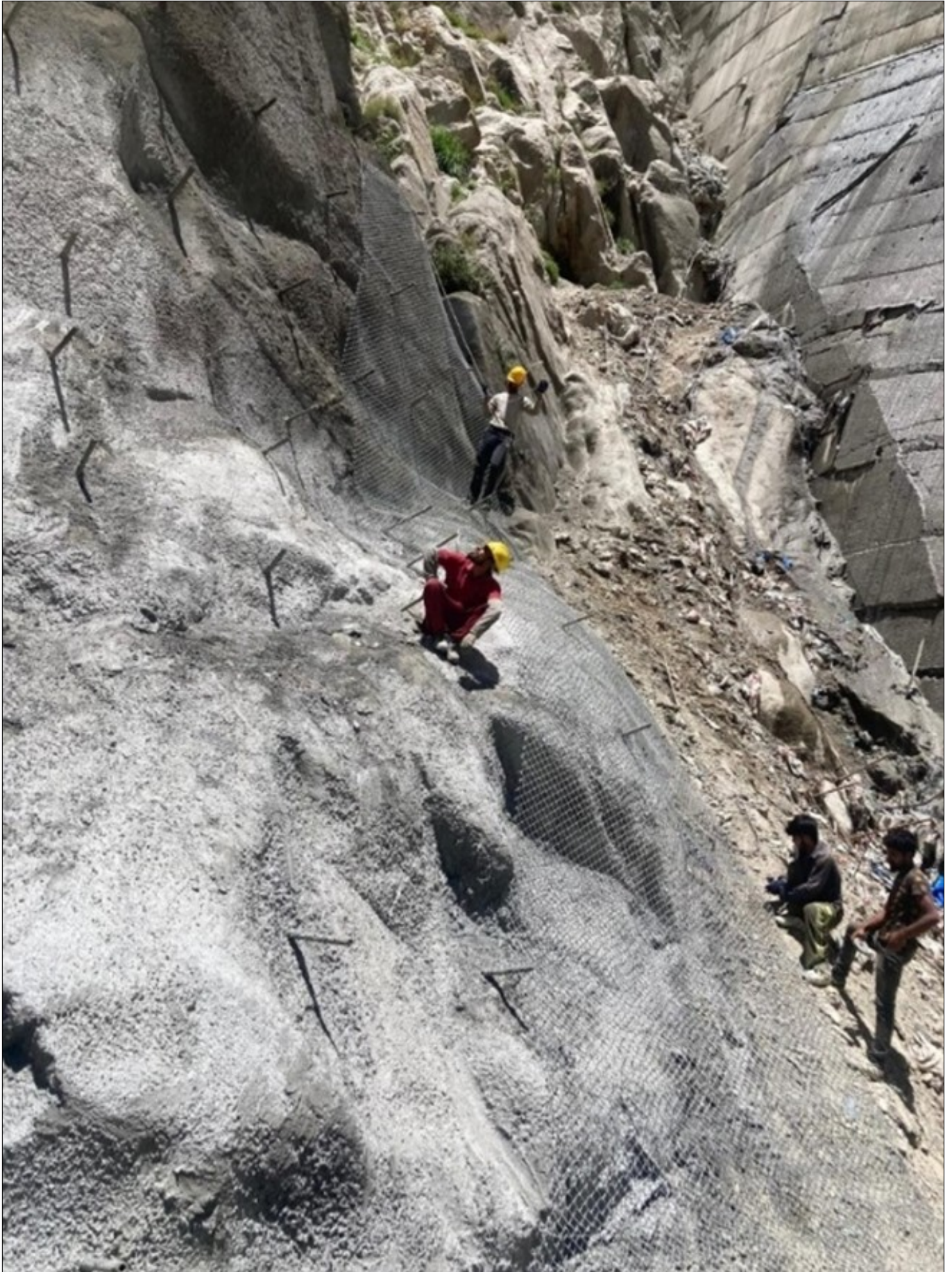
Photo 3 : During Construction Photograph
