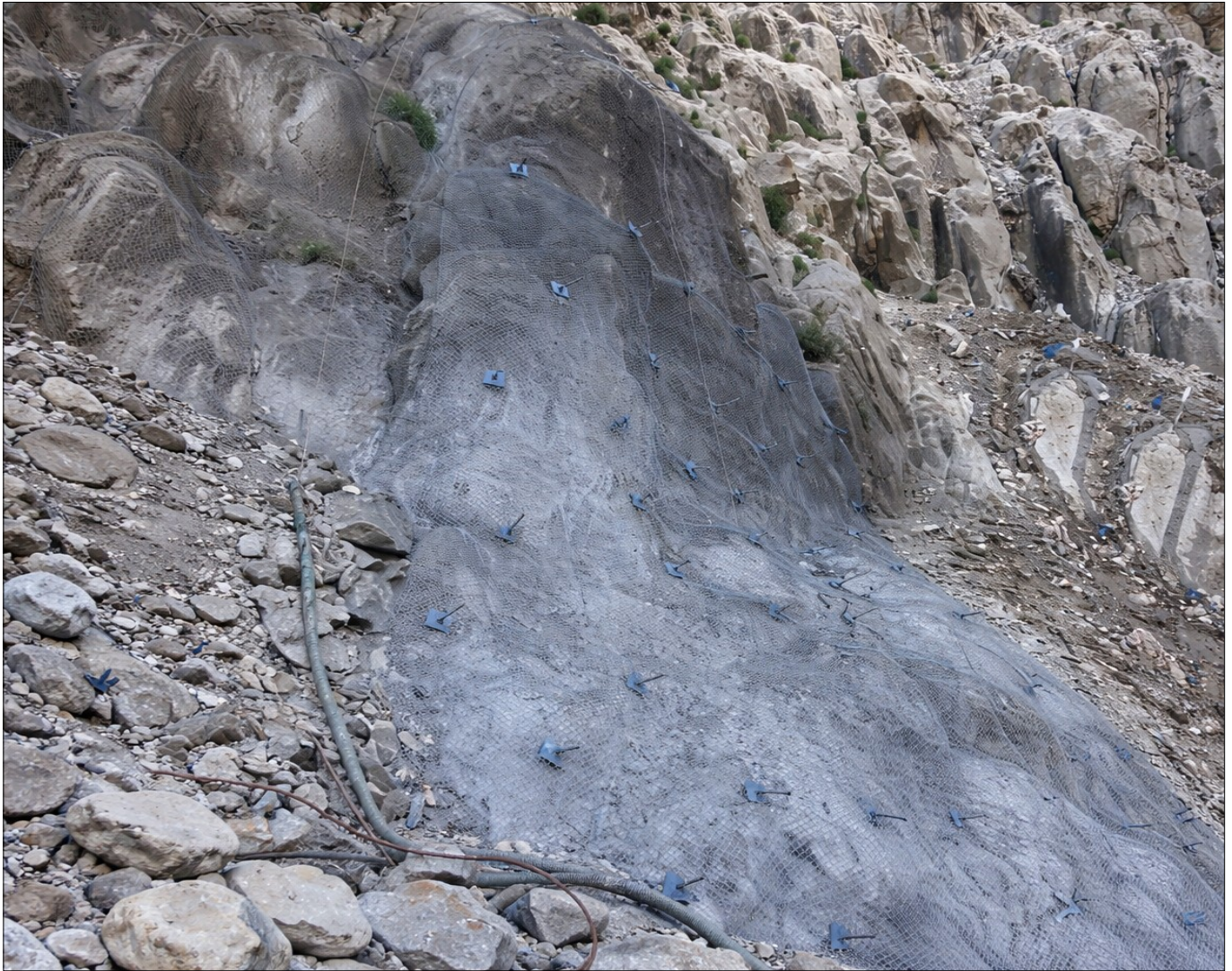
Photo 4 : Execution of Slope Stabilization Measures
