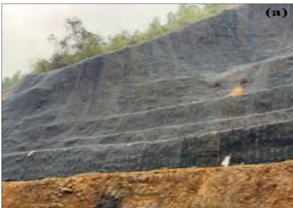
Photo 3 : During Construction Photograph
