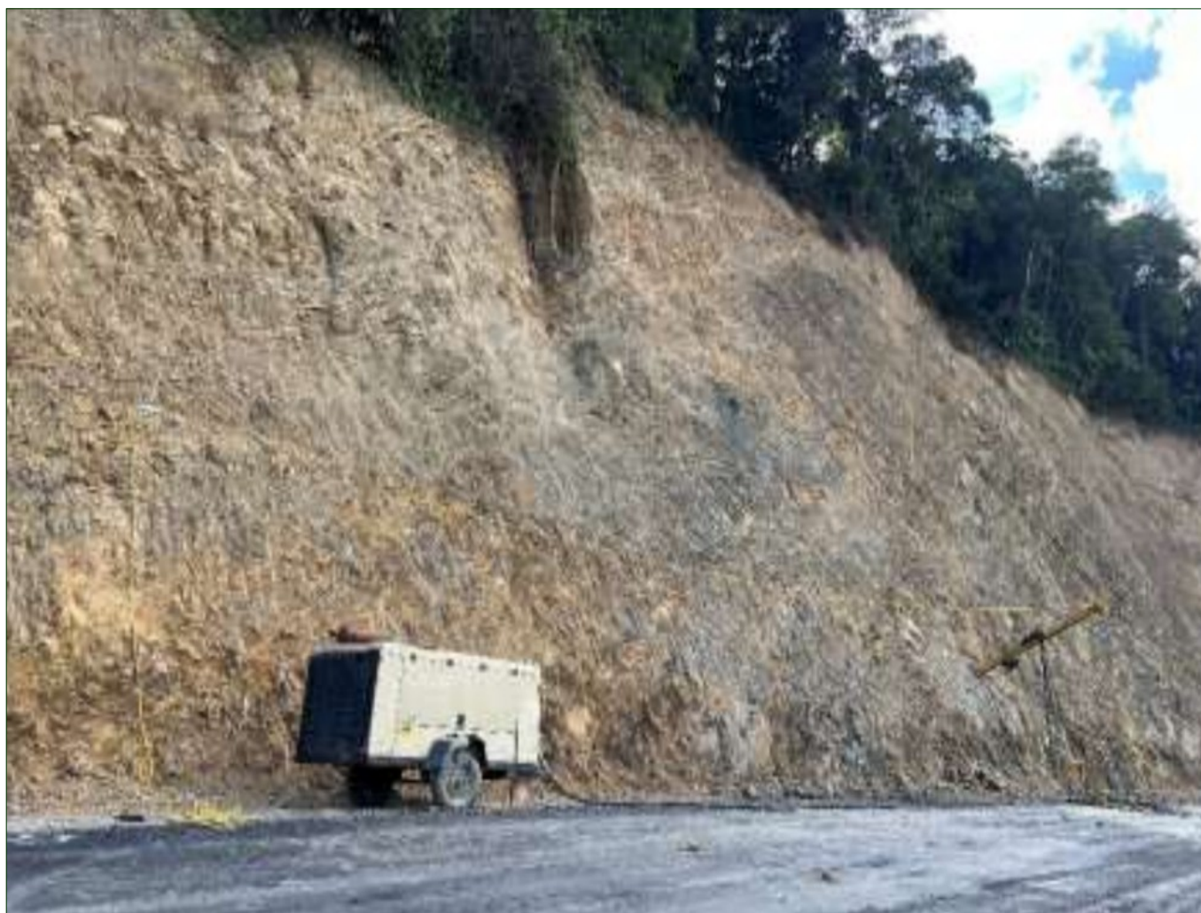
Photo 2 : Exposed Hill-side cut slope having weathered rock along package 9
