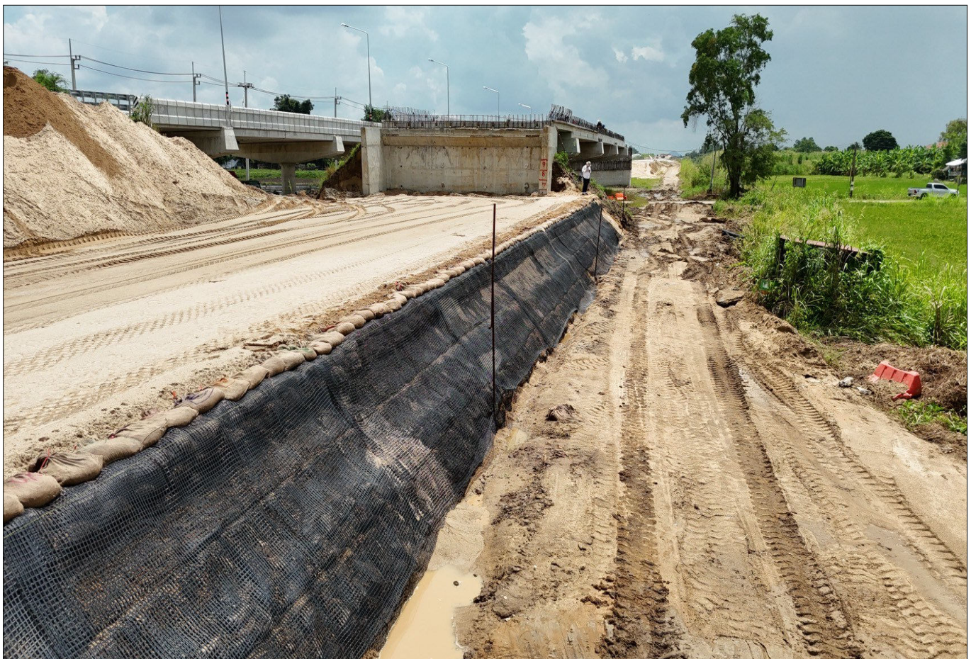
Photo 2 : TechGrid Geogrid Installation in Progress
