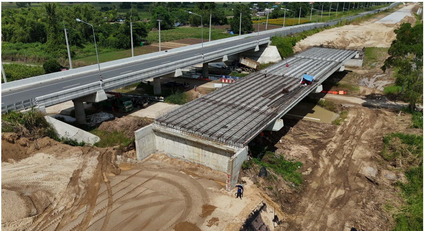
Photo 1 : Site Condition Before Reinforced Soil Embankment Construction
