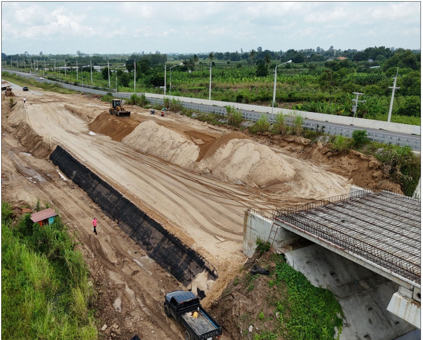
Photo 3 : During Construction photograph
